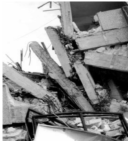
Figure 1.2: Typical Beam-Column Joint Failures (1999 Turkey earthquake) (Ghobarah et al; 2002)
