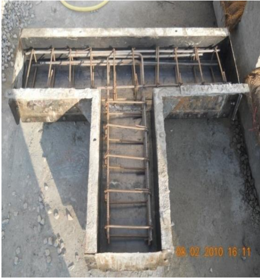
(c) Reinforcement Cage in Moulds
