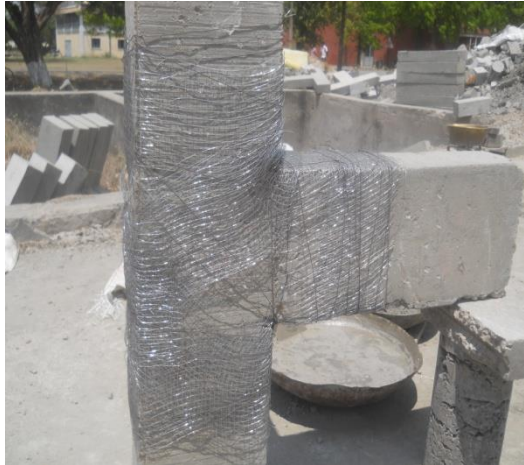
(a) Fixing of Wire Mesh
