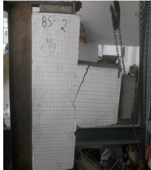
Crack Pattern in Four Layers Retrofitted Joint
