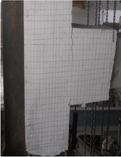
Crack Pattern in Two Layers Retrofitted Joint
