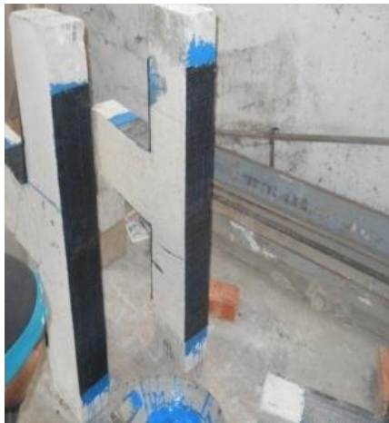
(a) Application of CFRP
