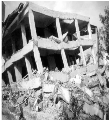
Figure 1.2: Typical Beam-Column Joint Failures (1999 Turkey earthquake) (Ghobarah et al; 2002)
