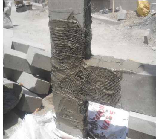
(b) Application of Cement Slurry
