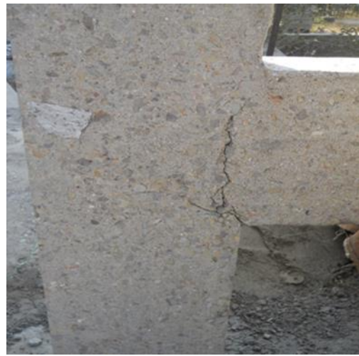
(b) Prepared Surface for Stress Level-2
