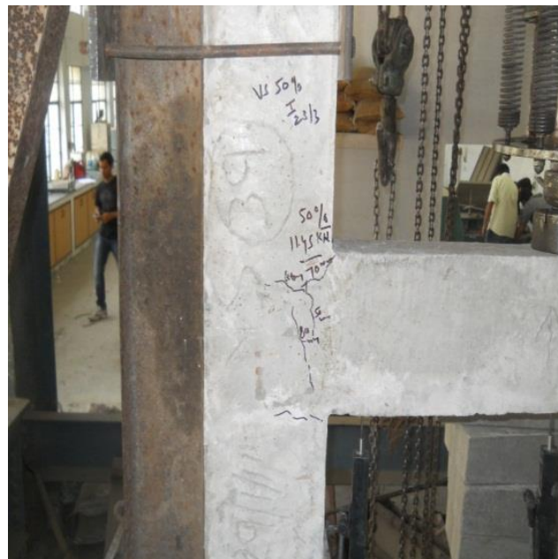
Plate 5.4: Crack Patterns in Control Beam-Column Joints Stressed to 50 Percent of Ultimate Load i.e. Stress Level-3
