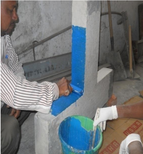
(c) Application of Epoxy
