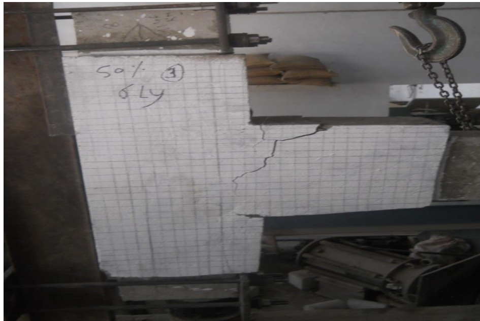
Crack Pattern in Six Layers Retrofitted Joint
