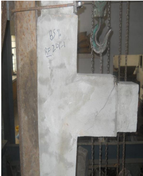
Crack Pattern in Two Layers Retrofitted Joint
