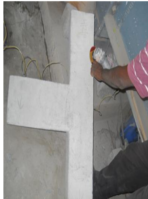
(b) Rounding of Edges
