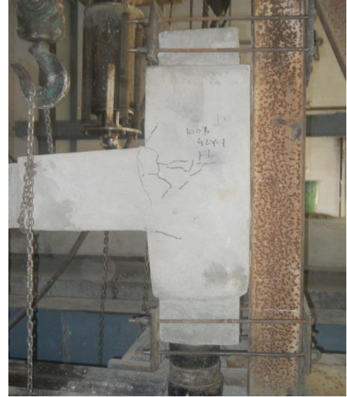
Crack Pattern in Four Layers Retrofitted Joint
