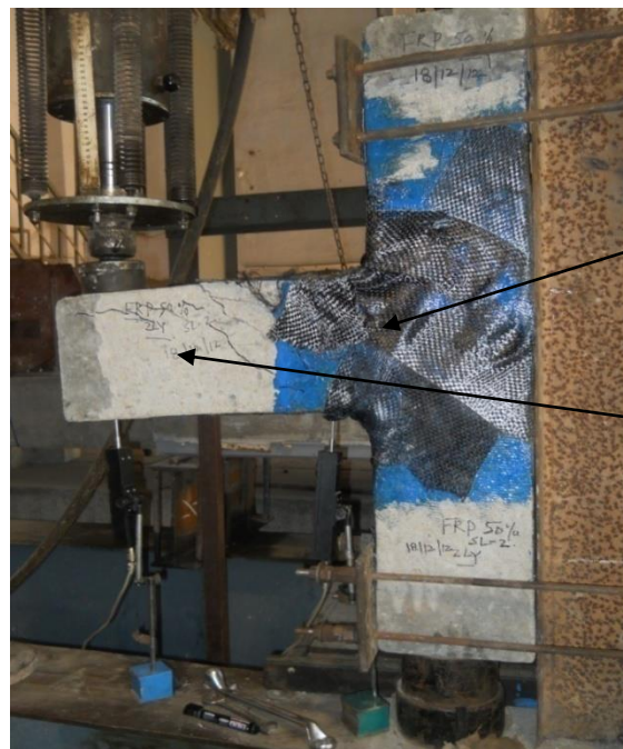
Plate 5.9: Failure of Beam-column Joints Retrofitted with CFRP Jacket with Two Layers for Stress Level-3
