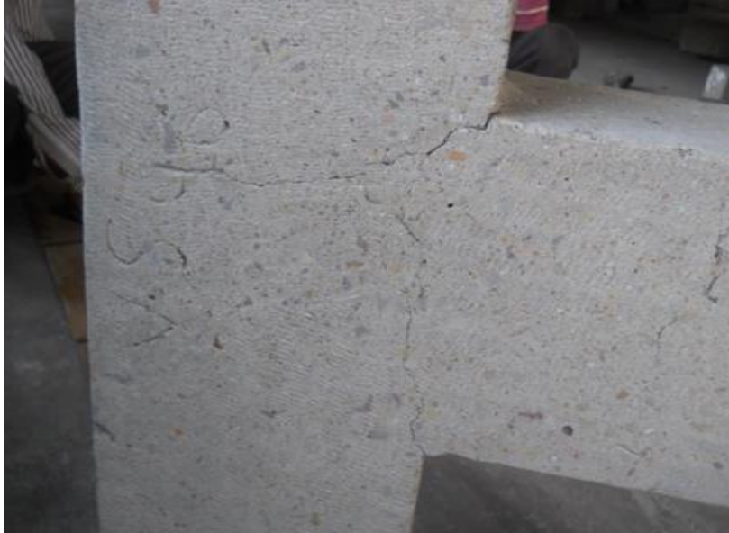
(c) Prepared Surface for Stress Level-3
