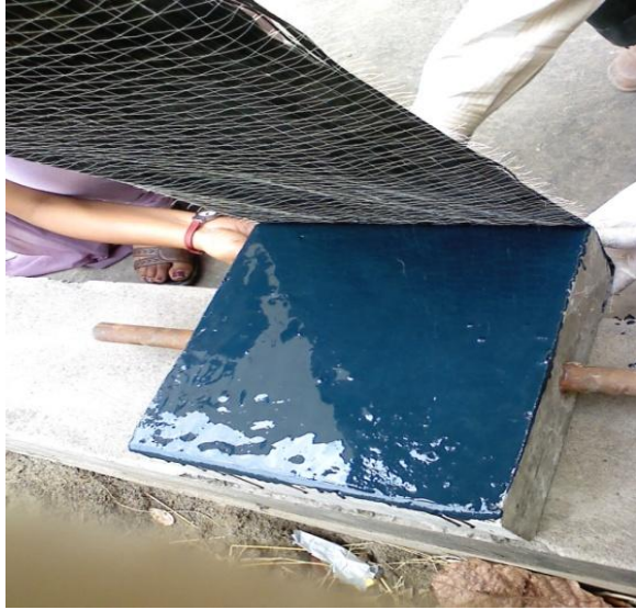
Fig 6.14 Placing Carbon Fiber Sheets
