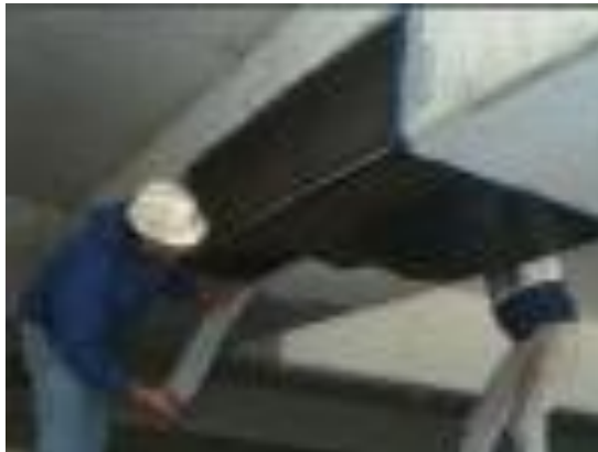
Fig.4.6 Retrofitting of beam by FRP Sheets
