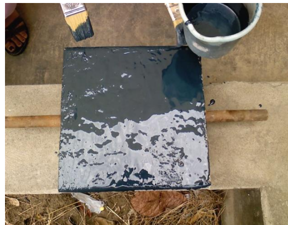
Figure 6.13 Applying Epoxy on Concrete
