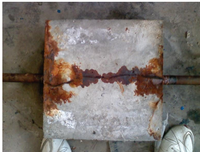
Fig. 7.3 Longitudinal crack along the length of rebar
