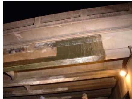
(b) FRP on a bridge structure
