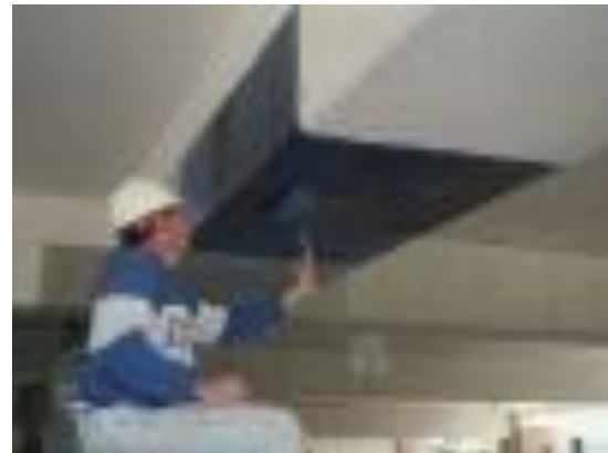
Fig.4.6 Retrofitting of beam by FRP Sheets
