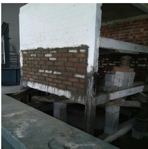
Figure 3.36 Brick infill after casting
