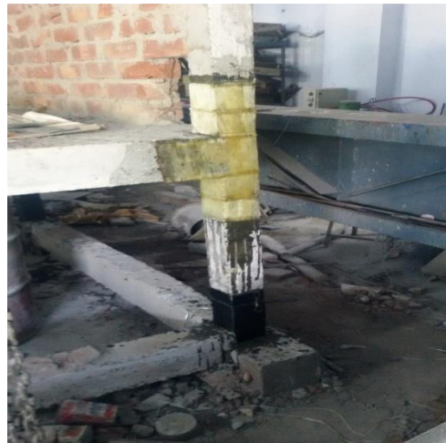
Figure 3.26 Final Retrofitted Frame
