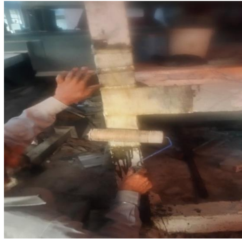
Figure 3.24 GFRP with M Brace epoxy
