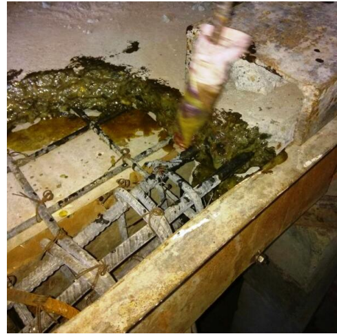
Figure 3.33 Epoxy applied at joints
