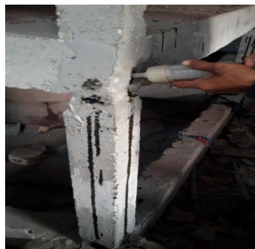
Figure 3.22 Injecting Master injector
