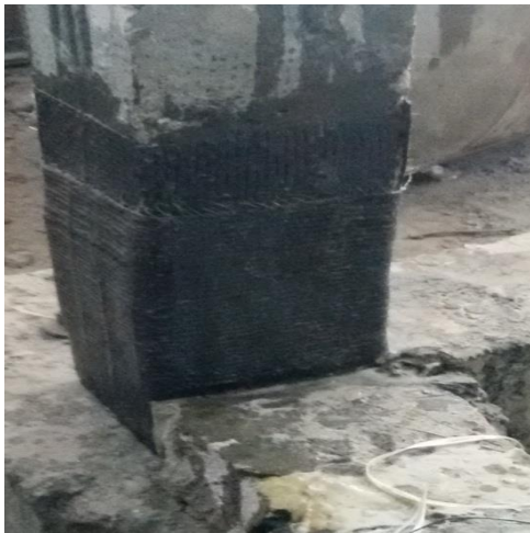
Figure 3.25 CFRP with M Brace epoxy
