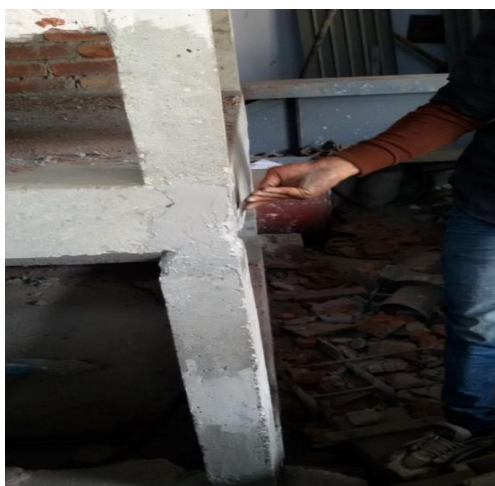
Figure 3.21 Void filling with M Brace putty
