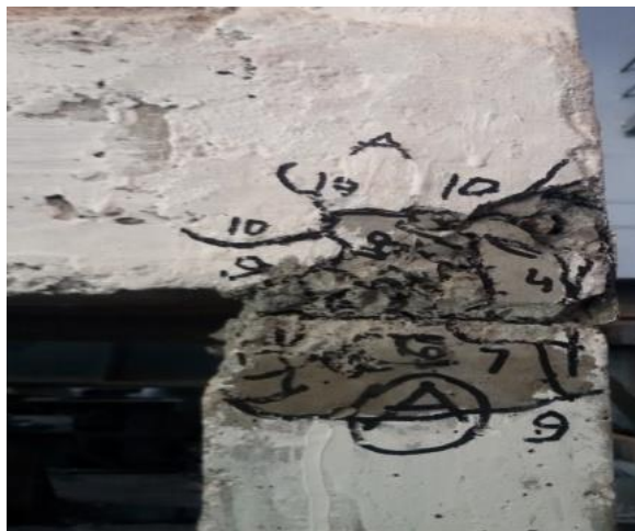
(a) Column-beam joint in A
