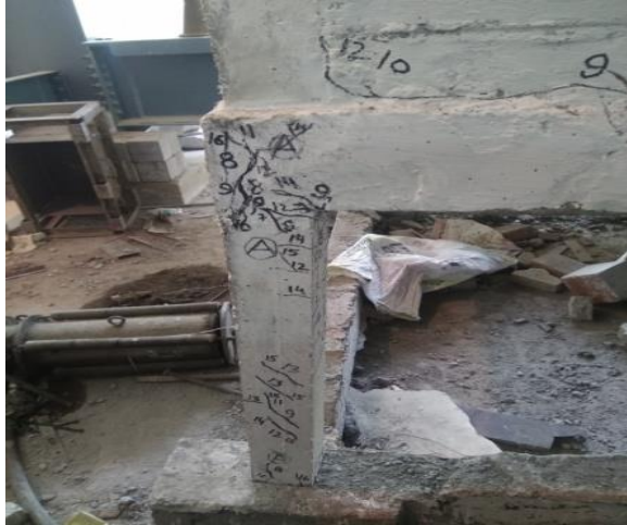
(a) Beam-Column Joint A
