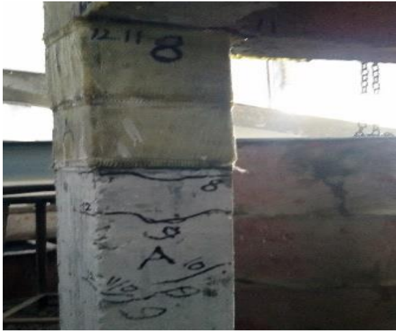
(e) Beam-Column Joint A
