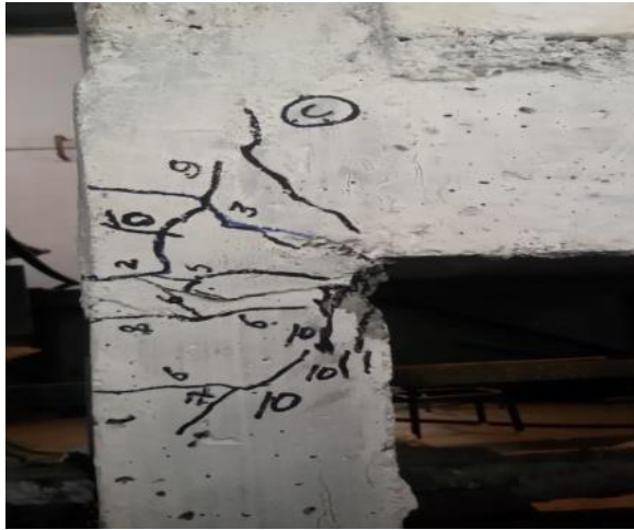
(c) Column-beam joint in C
