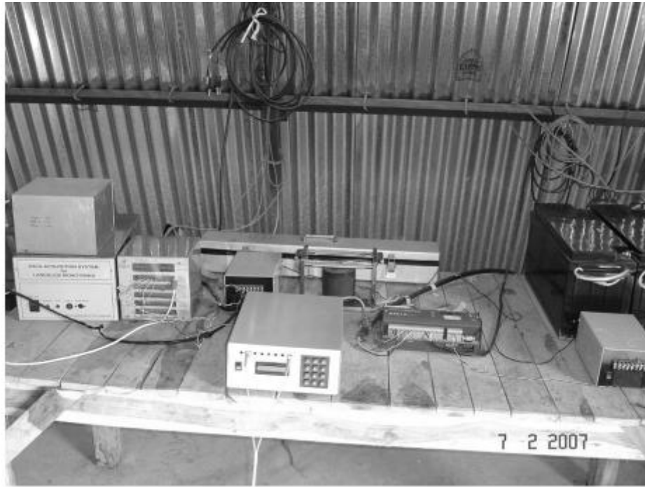
Figure 7.3 Installation of FBG Interrogator
