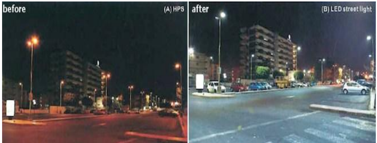
Figure 4.1: Night time lighting view of the HPS and LED lamp of different rating
