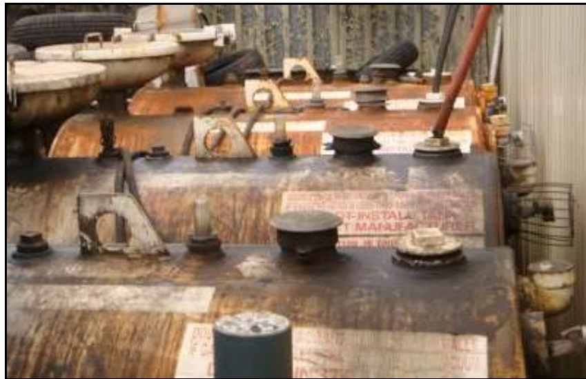
Figure 4.16: Transfer oil method: Fully Automatic
