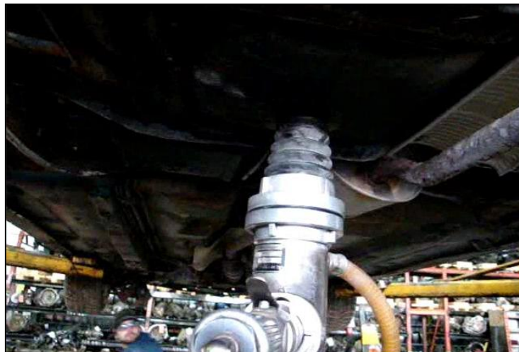
Figure 5.5: Drill for fuel tank
