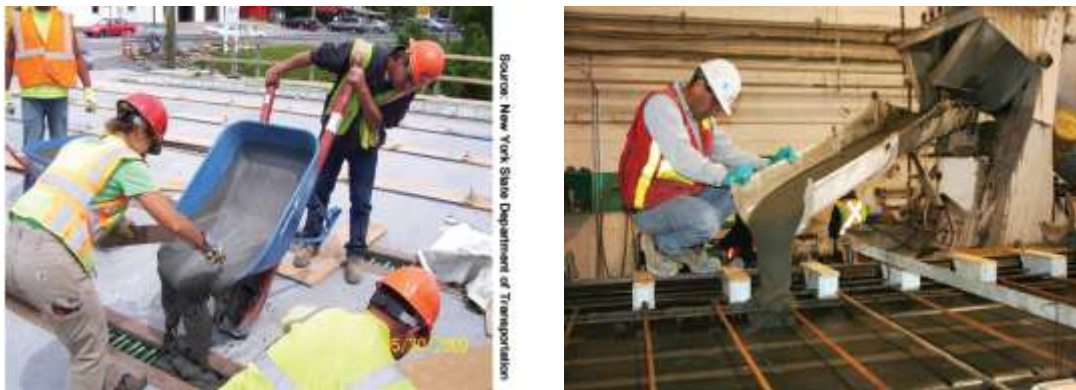
FIG. 2.9: Placing of UHPC
