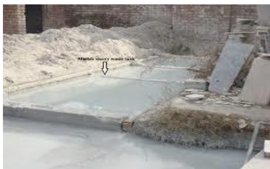
(c) Sedimentation tanks used for settlement of coarser marble particles
