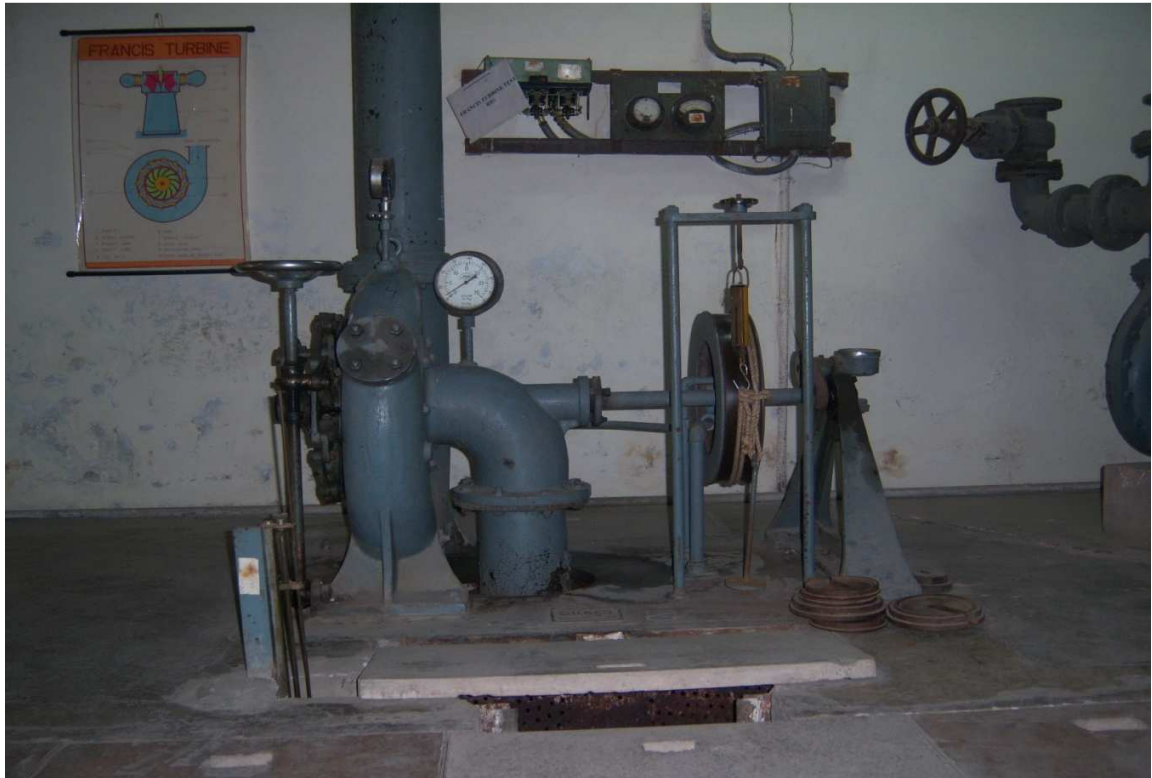
Fig 6.6 An overview of turbine set up used in experiment
