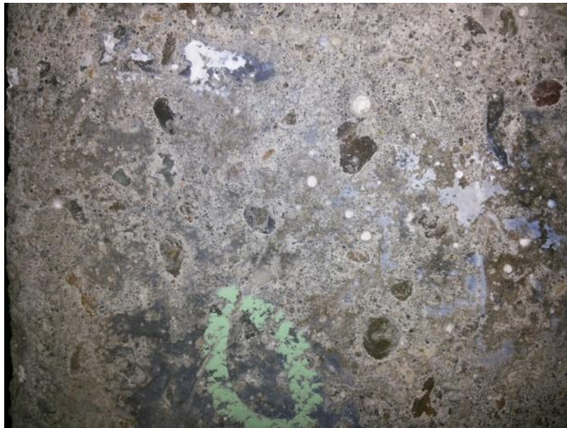
Fig. 3.12: Control concrete specimens after 365 days period of immersion in 10% magnesium sulfate solution (Concrete 'A')
