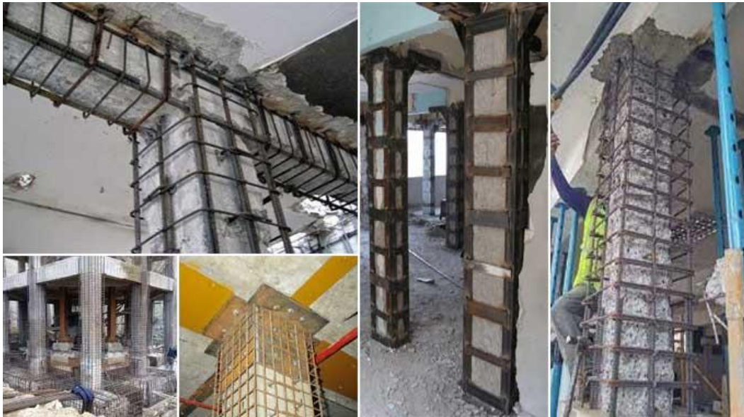
Fig.1.3 Different Retrofitting Techniques (Ref: www.tutorialtipscivil.com )
