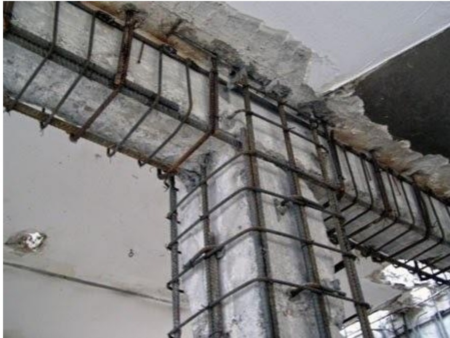
Fig. 1.5 Jacketing of Column and Beam (Ref: www.tutorialtipscivil.com )
