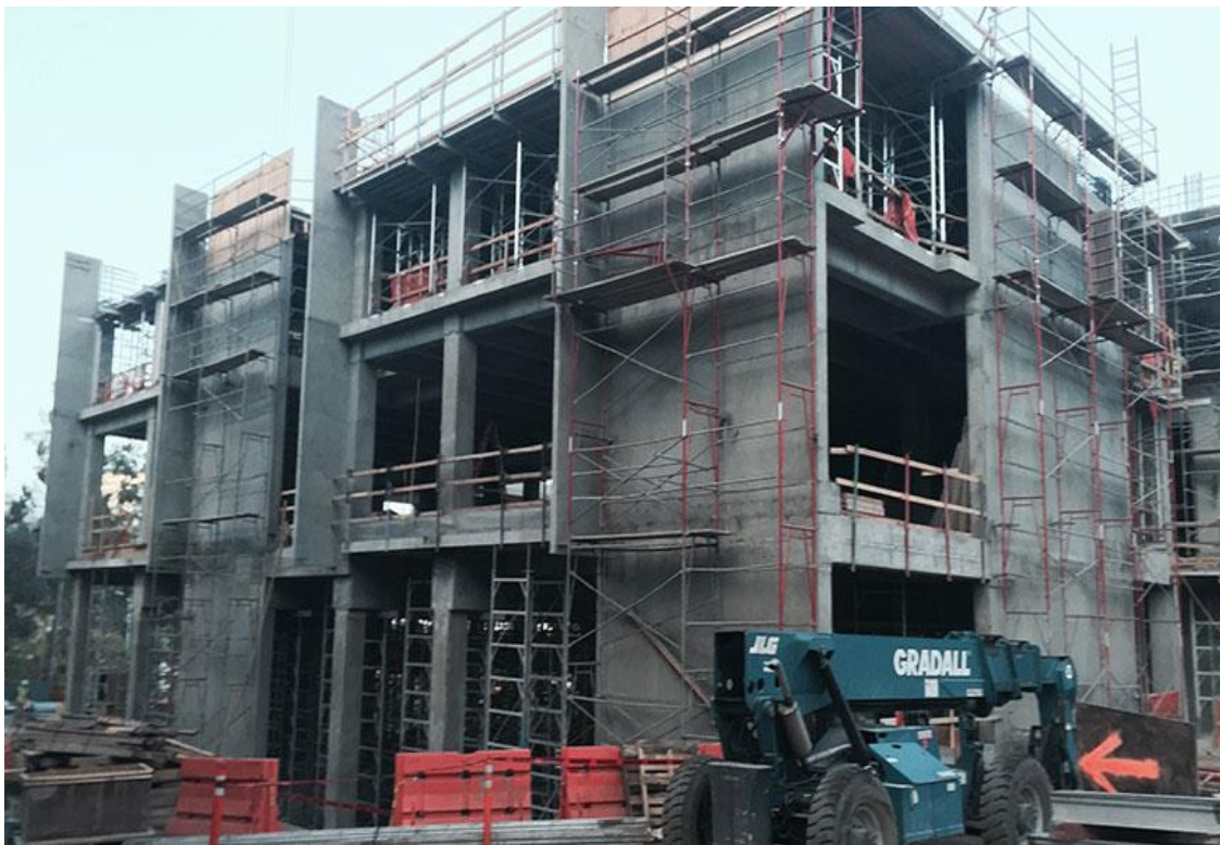
Fig. 1.9 Depiction of Shear Wall in a live project (Ref: www.tutorialtipscivil.com )
