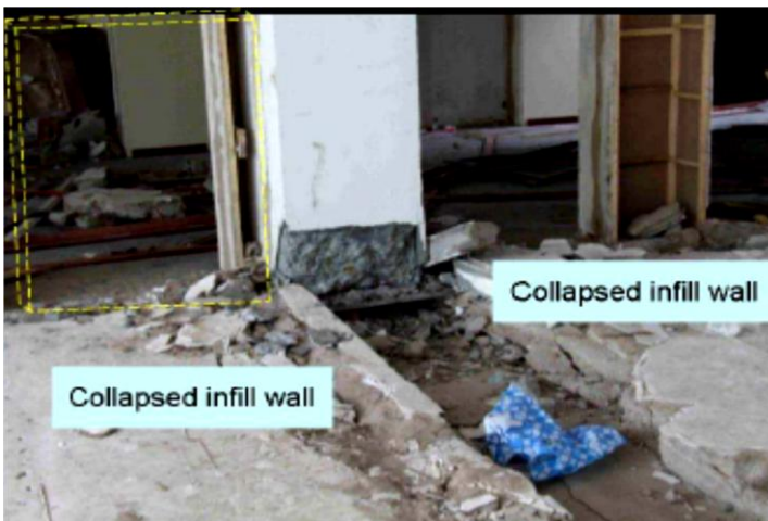
Fig-2.4, In-plane and Out plane failure of masonry infill. (Bixiong, Li et al.(2008)
