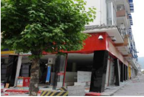
Fig 2.1(a) Overstressing of RCC frame.
