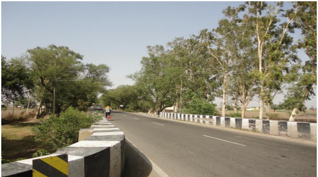
Narrow Bridge Along NH-64
