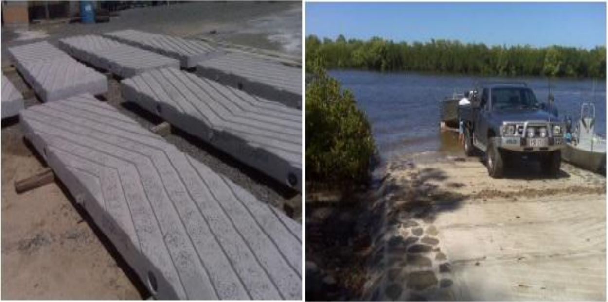
Fig.1.12: Boat ramp constructed with geopolymer concrete (Aldred and Day, 2012)
