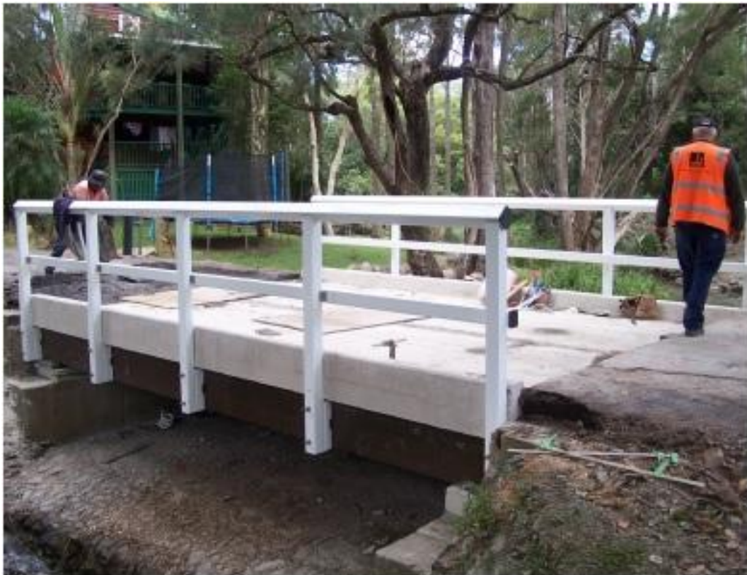
Fig.1.14: Composite girder and geopolymer concrete Deck Bridge in Brisbane (Aldred and Day, 2012)
