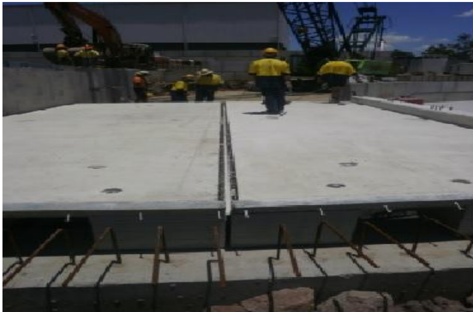
Fig.1.13: Installation of pre-fabricated geopolymer concrete bridge at Murrarie (Aldred and Day, 2012)
