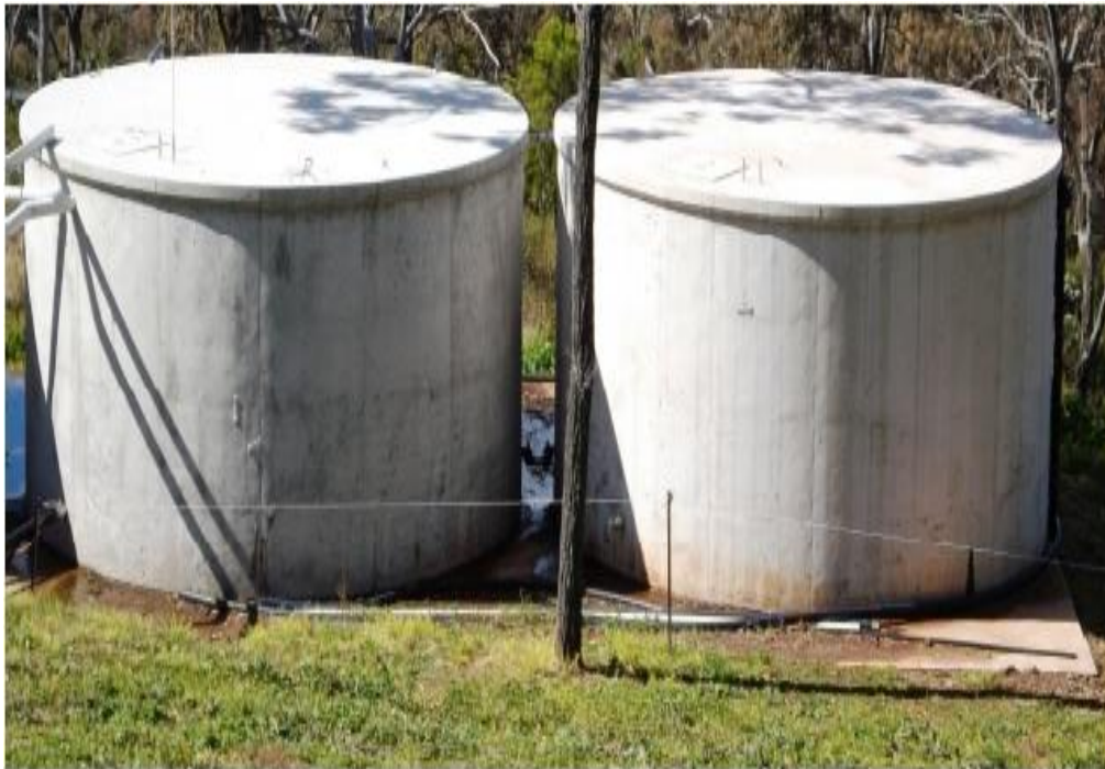
Fig.1.11: Water tanks cast with blended concrete (left) and geopolymer concrete (right) (Aldred and Day, 2012)
