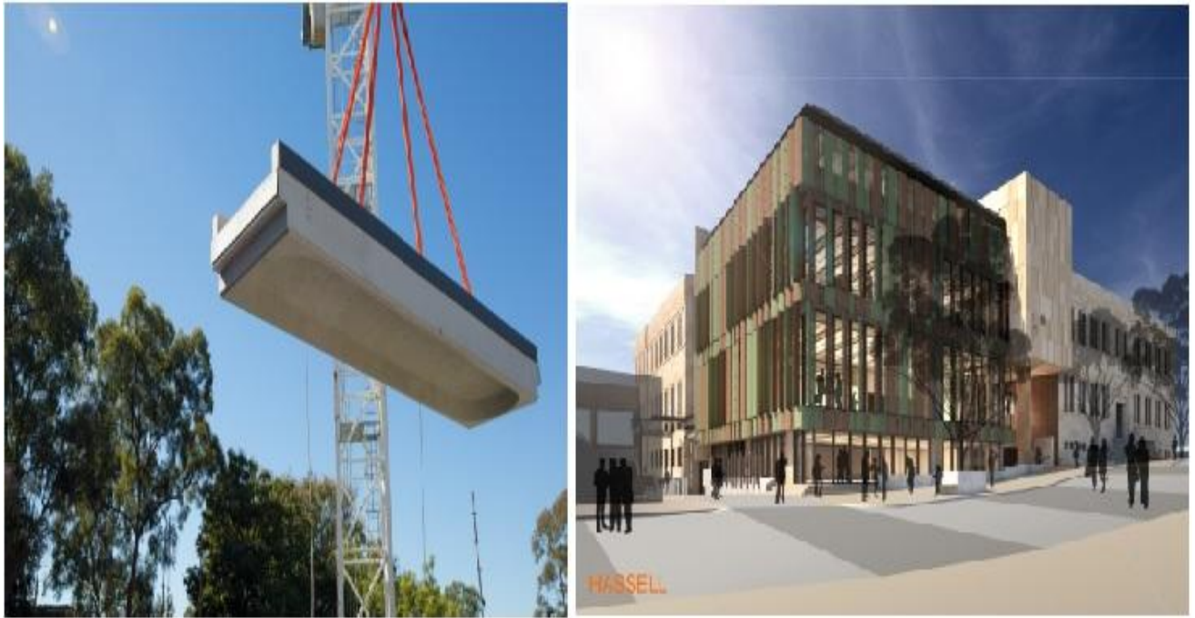
Fig.1.15: Geopolymer concrete floor beam (left) and rendered view of proposed building (right) (Aldred and Day, 2012)
