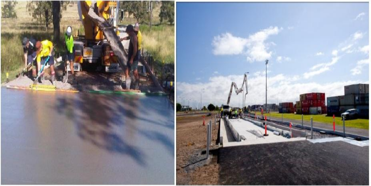
Fig.1.9: Placing of pavement using geopolymer concrete (Aldred and Day, 2012)
