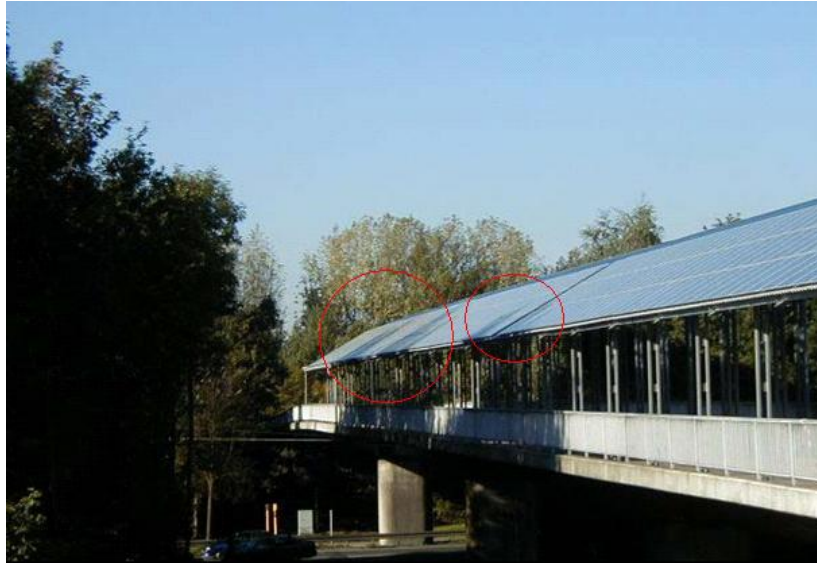
Figure (2.2) effect of shadow on PV modules.
