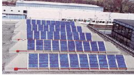
Figure (2.3.1) Flat roof system.
