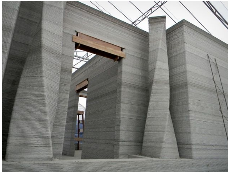
Fig 1.1: 3D printed concrete structure without formwork
