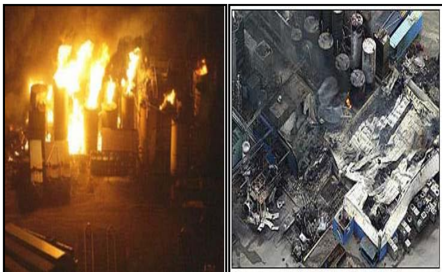
Fig: 2.3 : Photographs during and after the 2005 EQ Romulus fuel blending fire.
