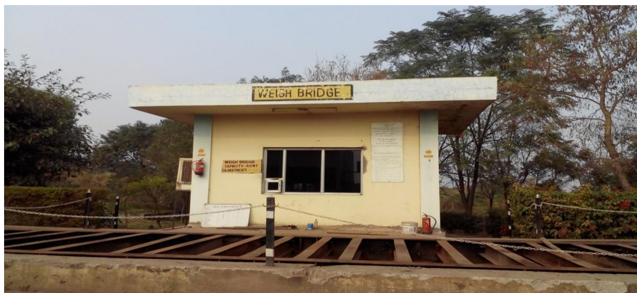
Figure- Weighing bridge
