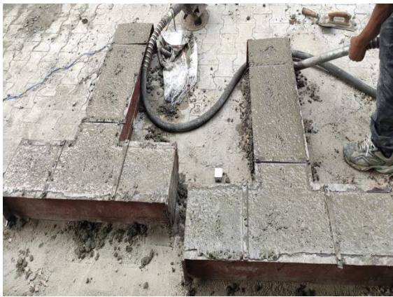
(c) Needle vibrator used for uniform vibration
