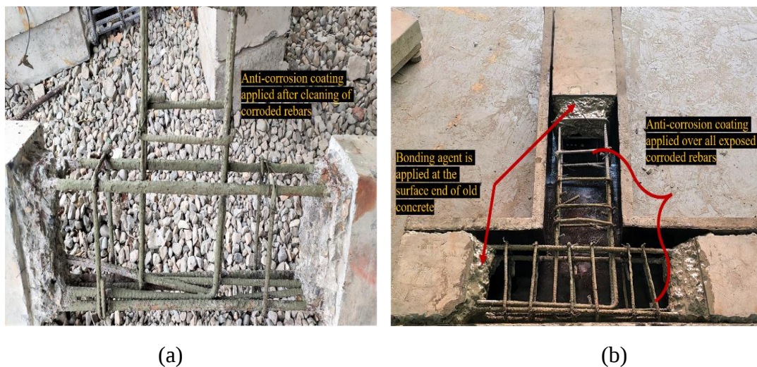
Figure 3. 25 (a) Application of anti-corrosive coating on the surface of corroded reinforcing bar, (b) Specimen placed in formwork for retrofitting
