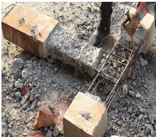
(a) Removal of corrosion damage concrete
