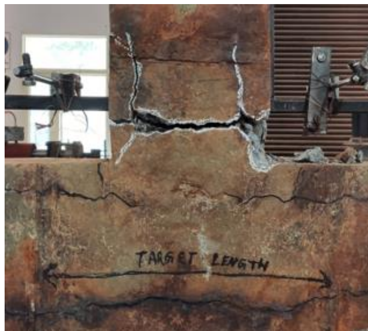
Figure 4. 10 Ultimate failure of NDC-3
