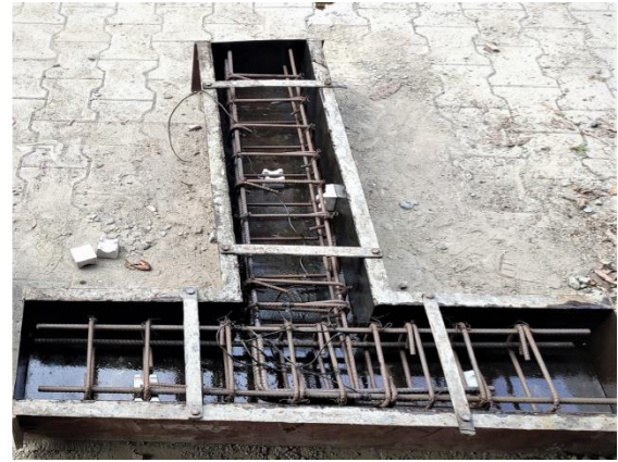
(b) Reinforcement cage inside the mould
