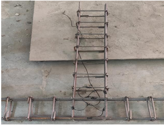
(a) Reinforcement cage
