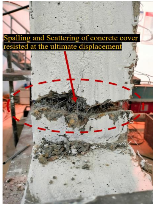
Figure 5. 11 Side view of the RD-3 specimen showing steel fiber-concrete bond
