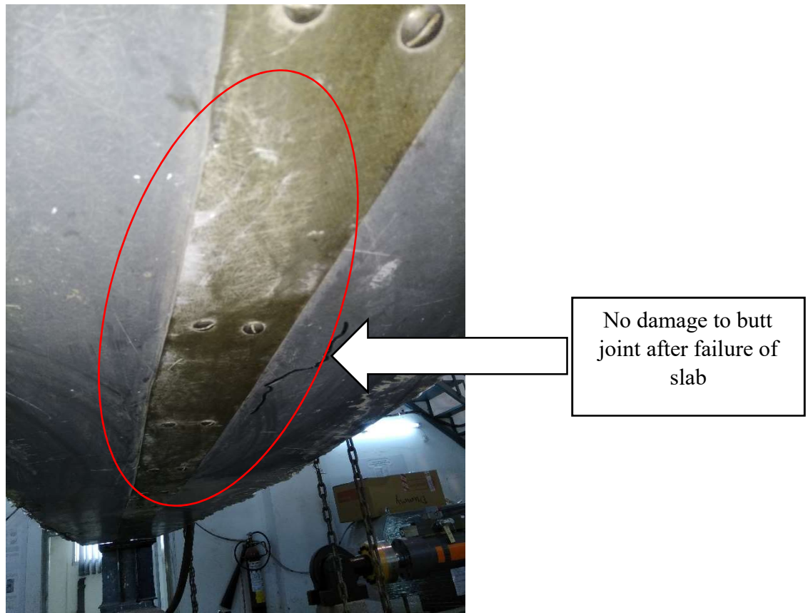
Fig 4.22 Condition of joint after failure of specimen SLB 0
