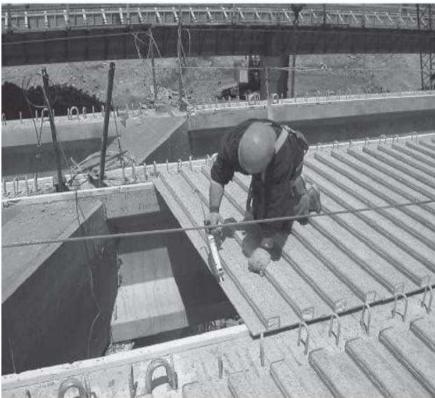
Fig.2.34. Installation of the CDS deck panels
