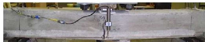
d) Flexural failure of specimen C1
