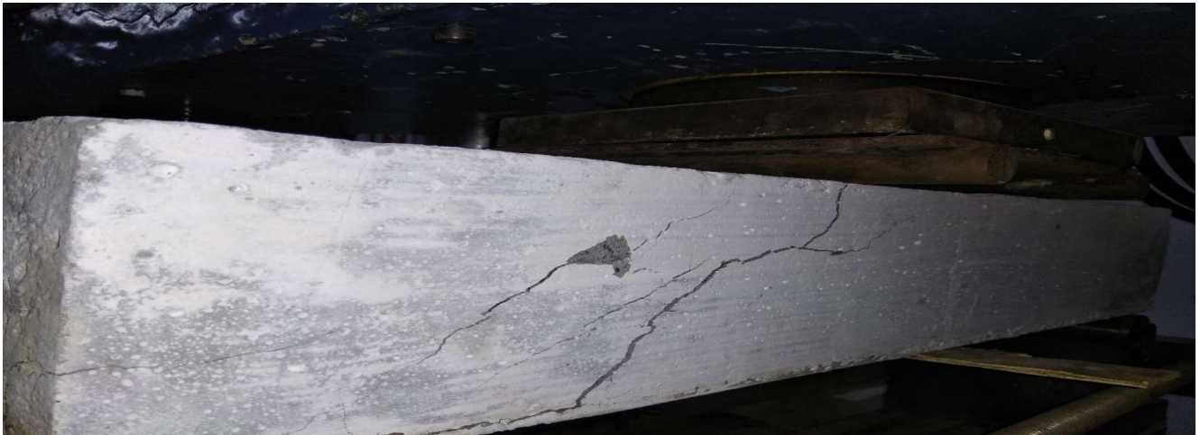
Fig 4.4 Shear failure in Control Beam
