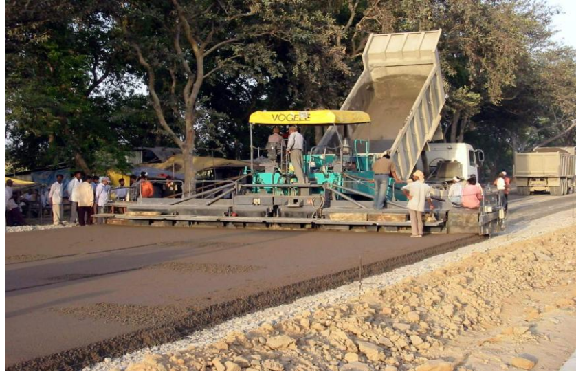
Fig 1.1 Pavement Dry Lean Concrete
