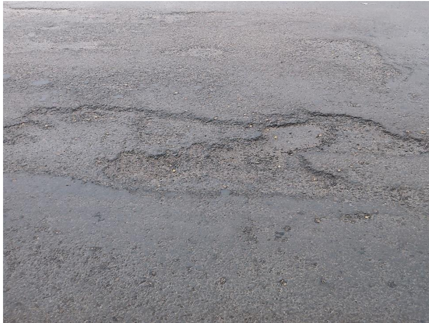
Fig. 3.17: Ravelled Surfaces
