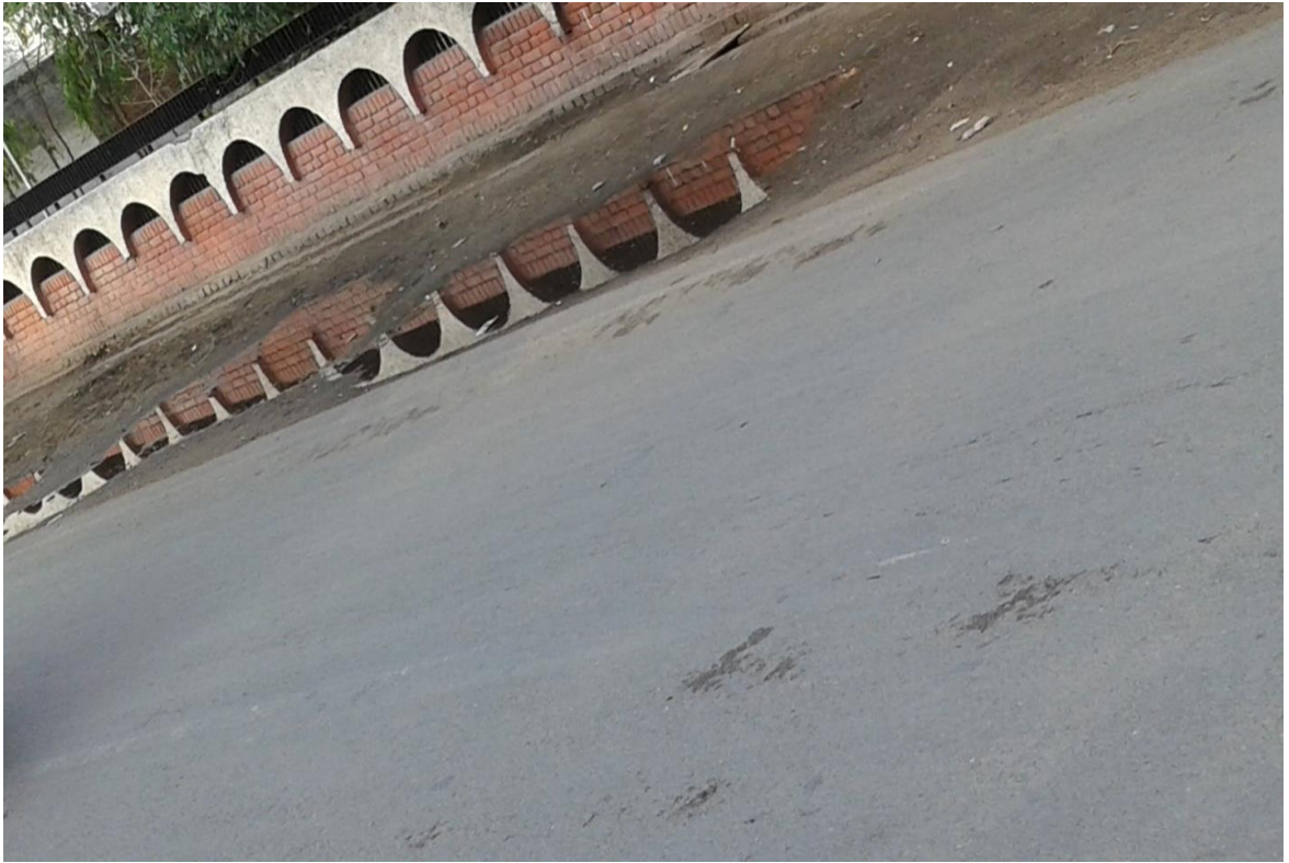
Fig. 3.5: Water on Shoulder side of Road Section UR02
