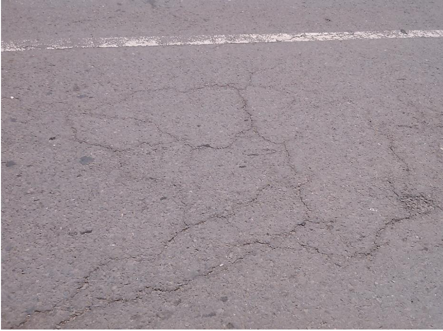
Fig. 3.15: Cracked Surface
