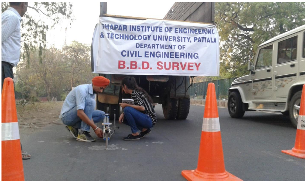
Fig. 3.9: BBD Test in Progress at Chainage 0.200 km, Section UR02
