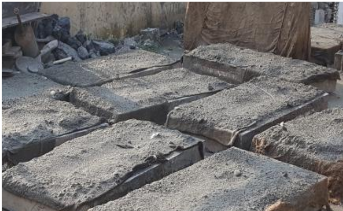
Figure 3.4 Curing of EPS sandwiched concrete panels
