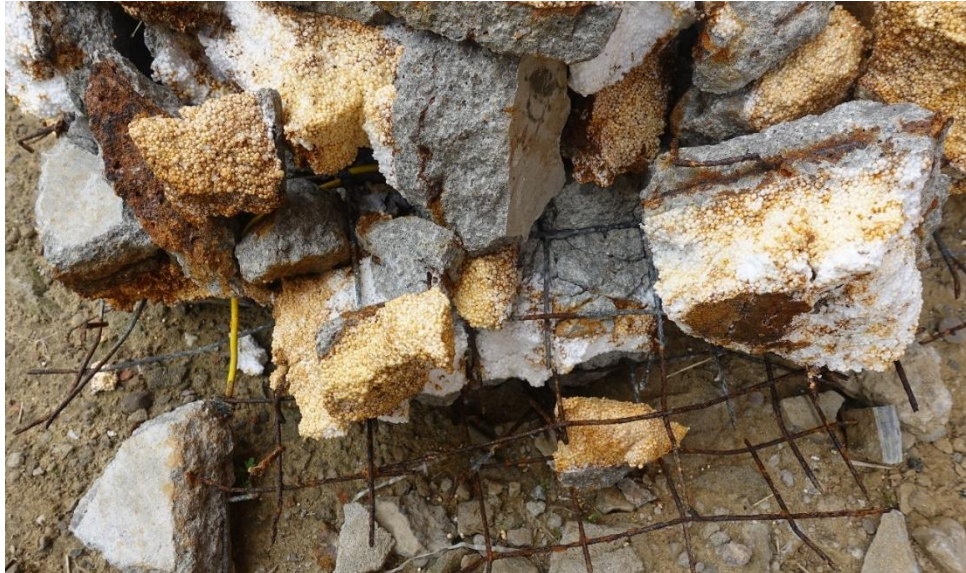
Figure 4.3 Extricated EPS and wire mesh after panel testing
