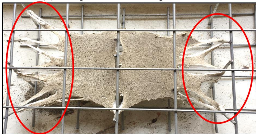
(c) EPS panel skeleton exposed to 120 0 C
