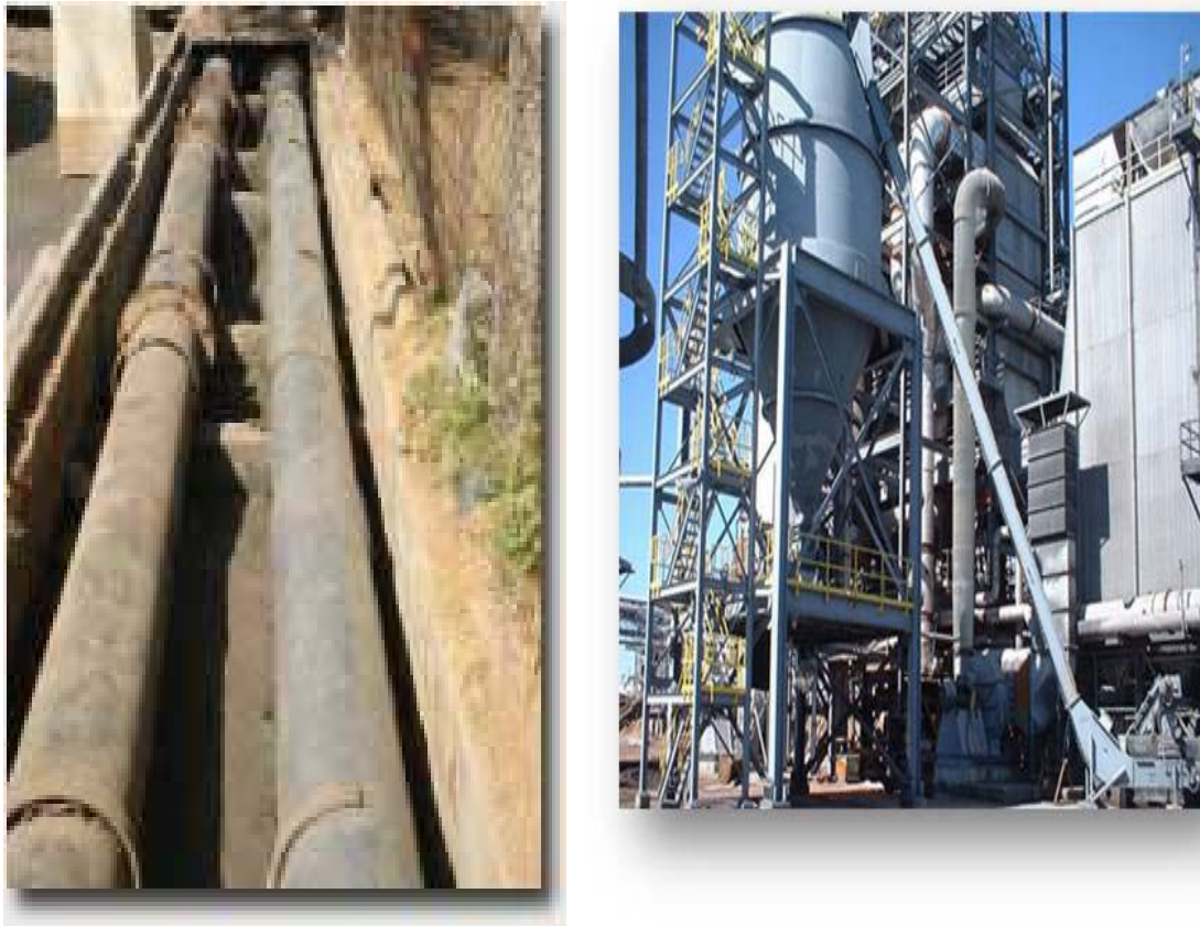
Figure 1.2 Ash slurry disposal systems
