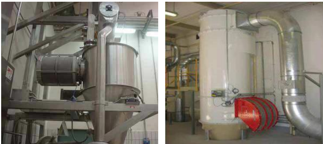
Figure 2.5: Flameless vents type and their use [13]
