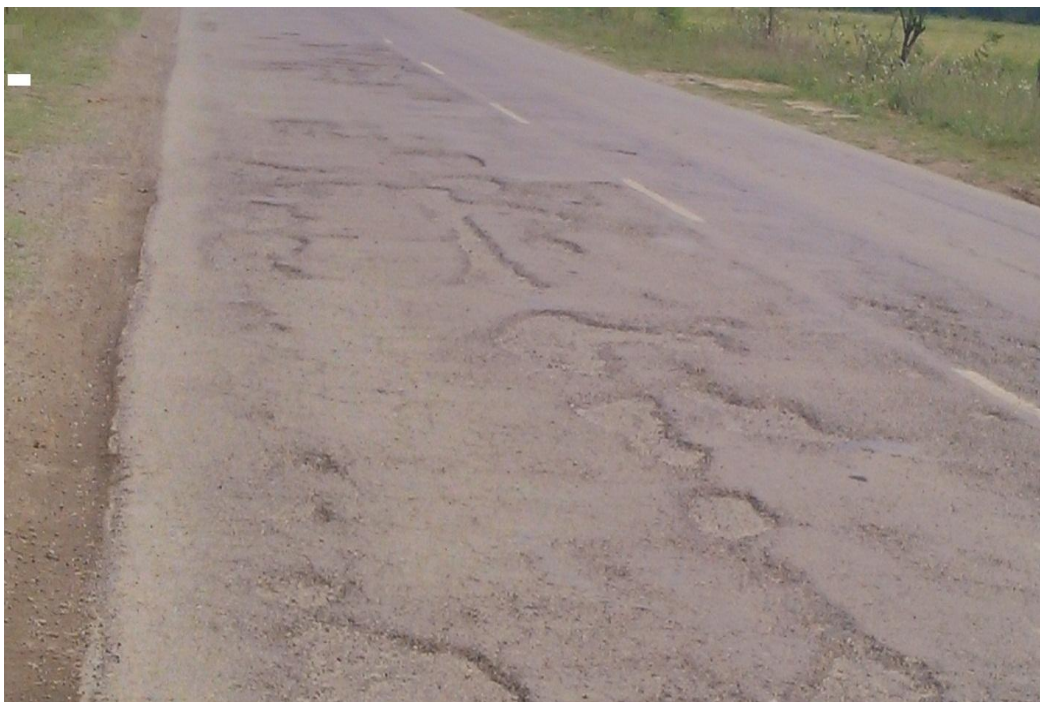
Fig 3.3: Cracking coupled with raveling at km 95.000
