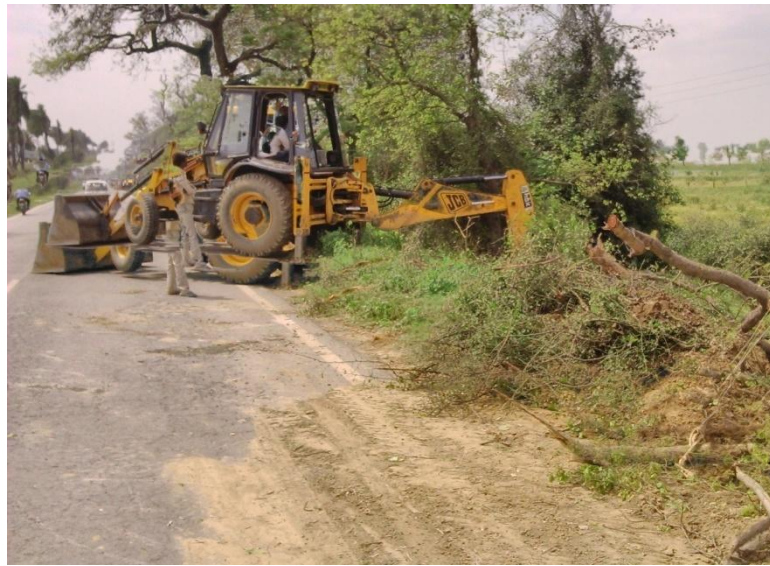
Fig. 5.6: Felling of trees along the road side
