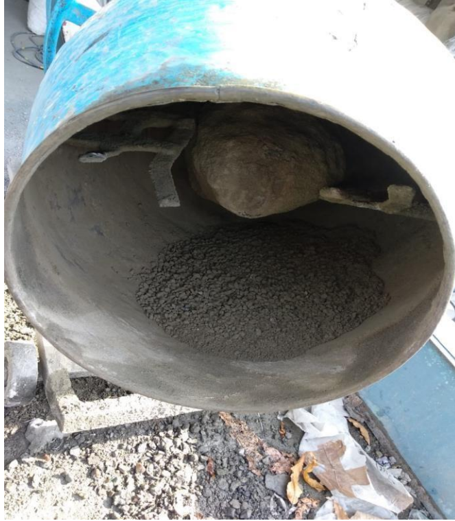
Figure 5.5: Round concrete mixer with dry ingredients
