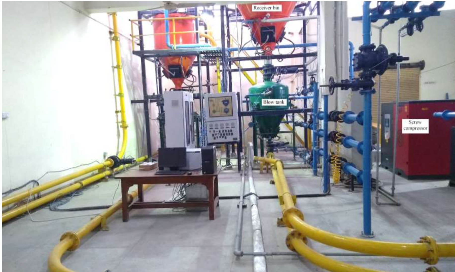
Figure 2.8: A part of the new large scale test facility
