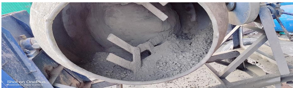
Figure 4-4 Dry mixing of Concrete.
