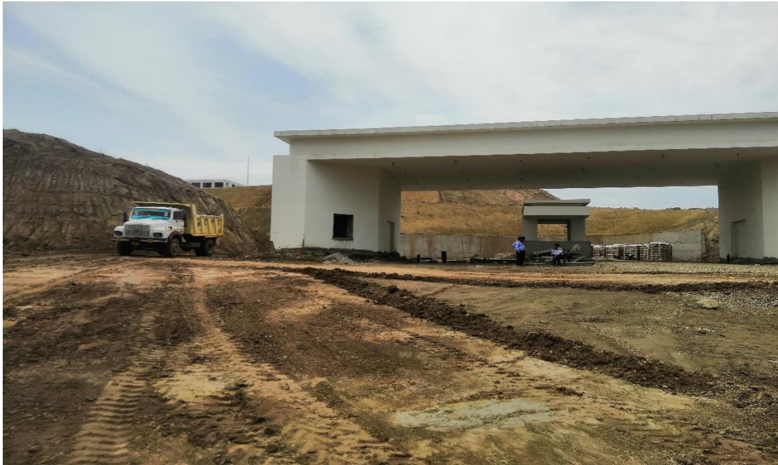
Figure 3.32: Front gate of IIM Jammu before construction
