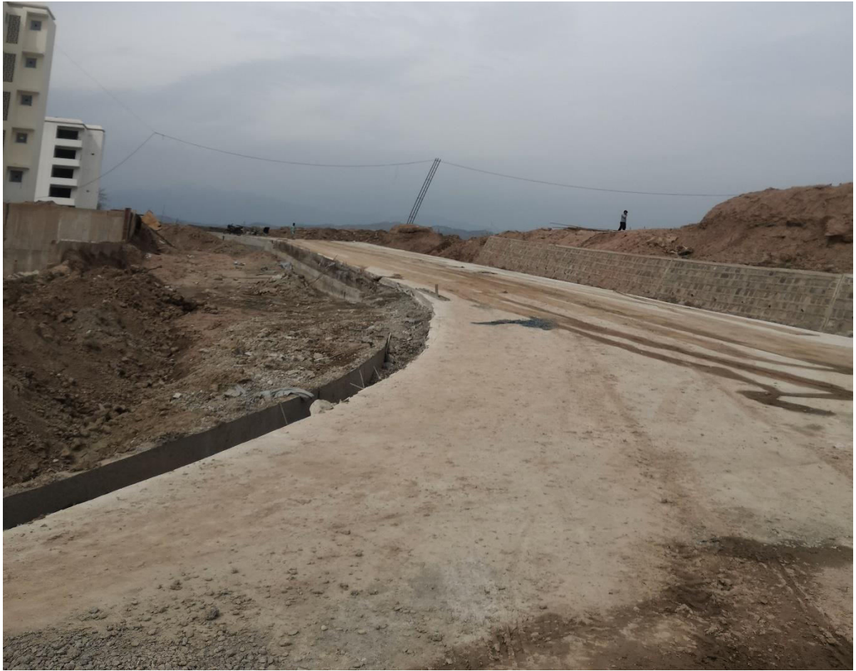
Figure 3.35: Site Photograph of MCW-05
