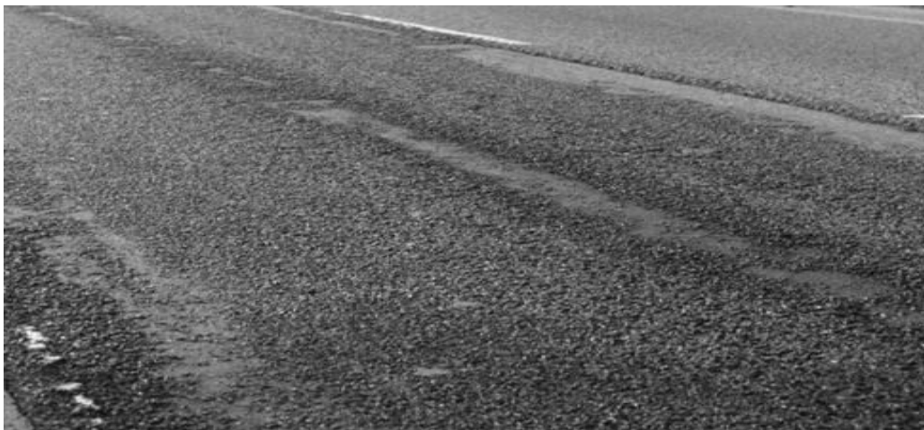
Figure 5.8: Raveling Representation
