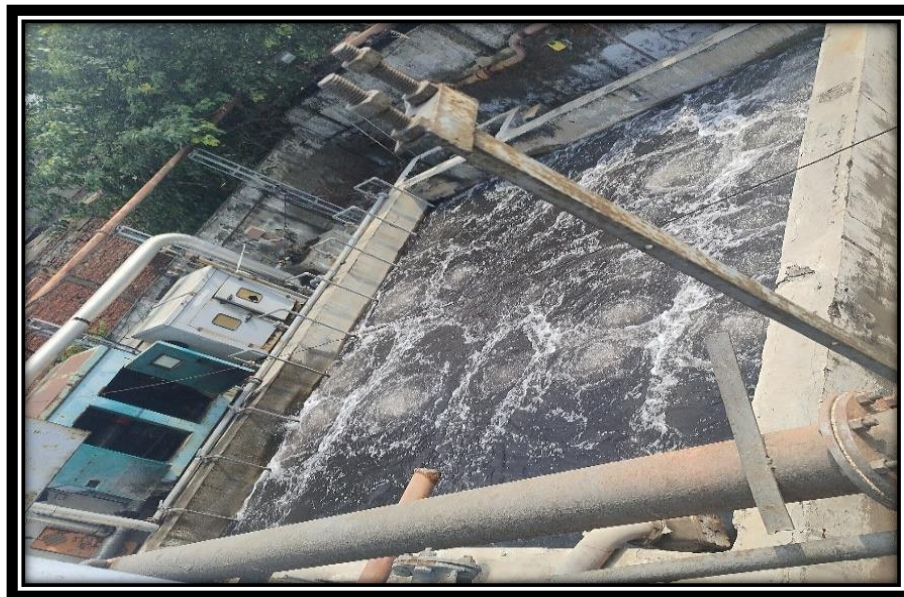
Figure 1.1: ETP (OCM Pvt. Ltd., Amritsar, Punjab) using conventional ASP
