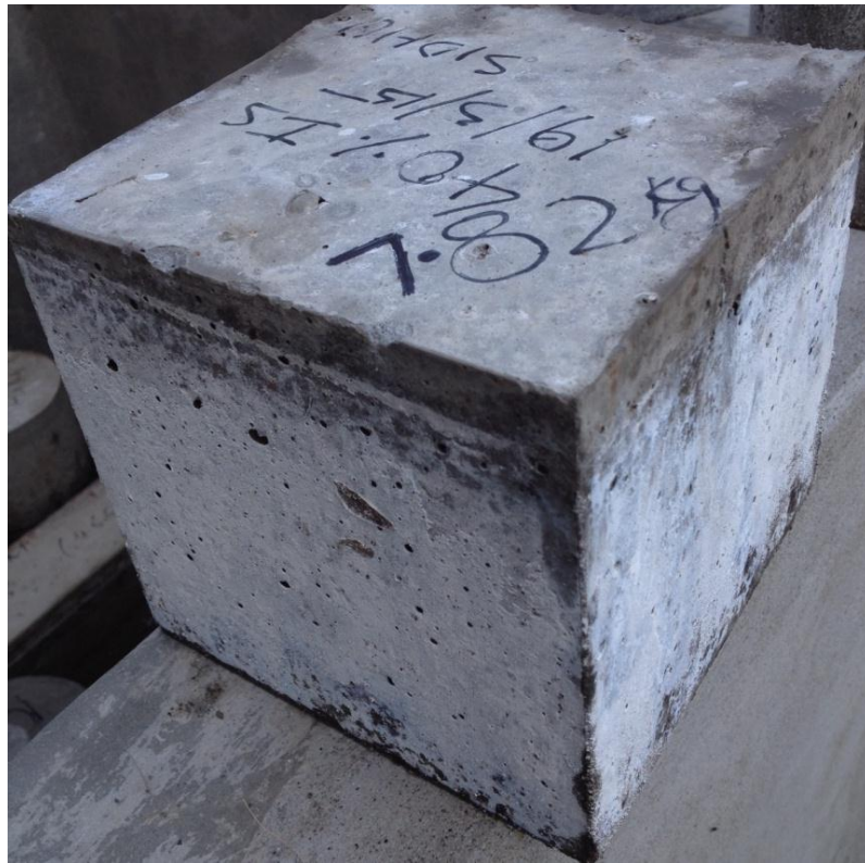
Fig. 3.17: SCC specimen after 365 days period of immersion in 10% magnesium sulphate solution
