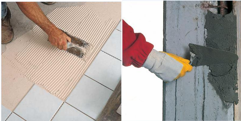
Figure 1.1 Application of Polymer Mortar in Flooring and Repairing
