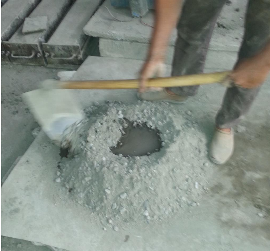
Plate 3.1: Concrete Mixture Preparation
