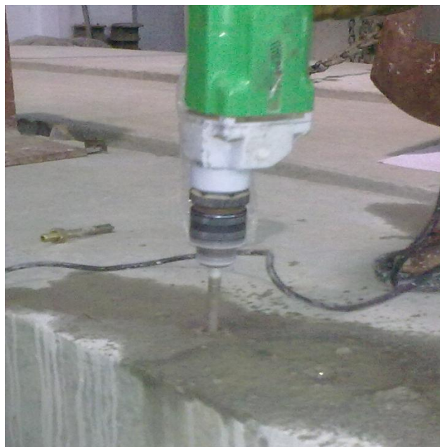
Fig 3.13: Drilling of holes for fasteners for anchoring the machine and plate on both sides of the beam.
