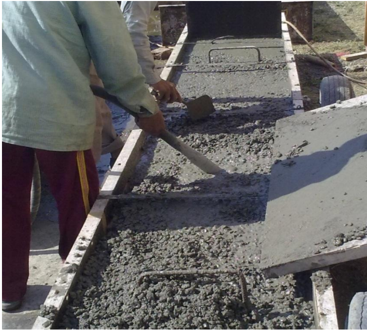
Fig 3.10: Use of vibrators for proper compaction
