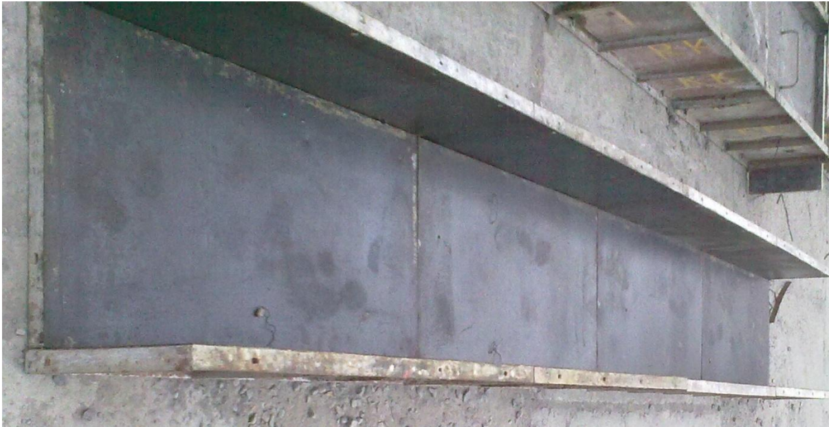
Fig 3.8: Formation of formwork by joining shuttering plates
