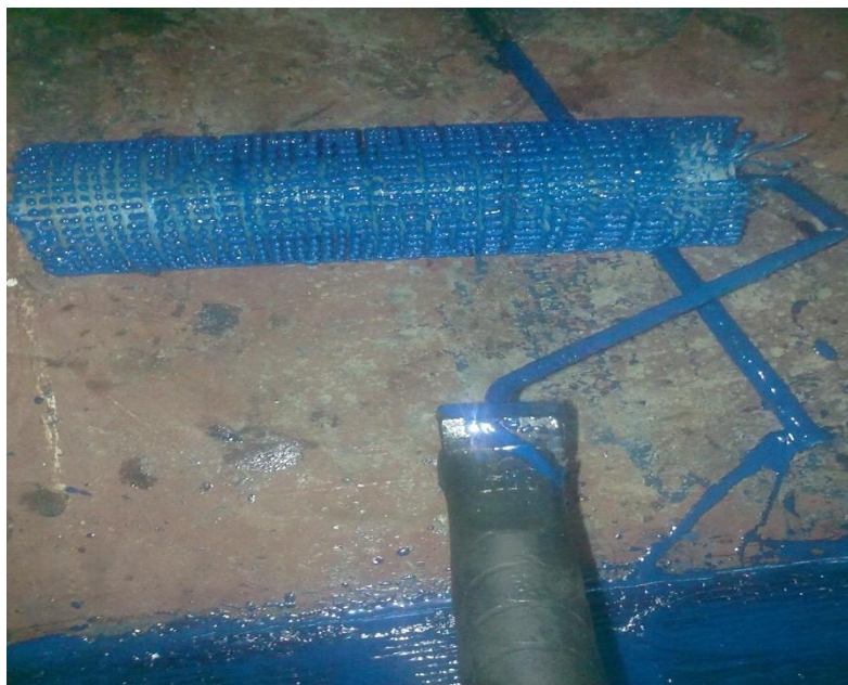
Fig 3.4: Roller for proper adhesion of saturant to fibre
