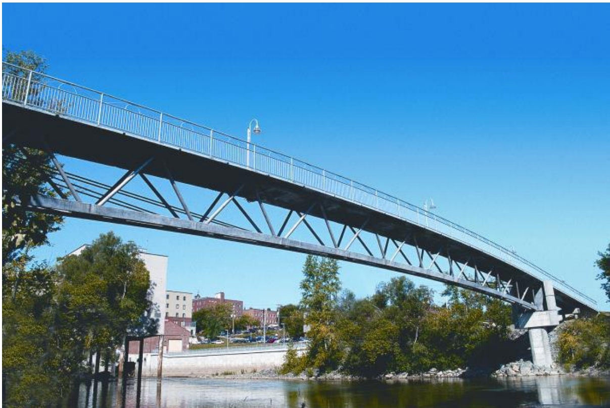
Fig.1.9: Sherbrooke footbridge [Karmout, M; 2009]
