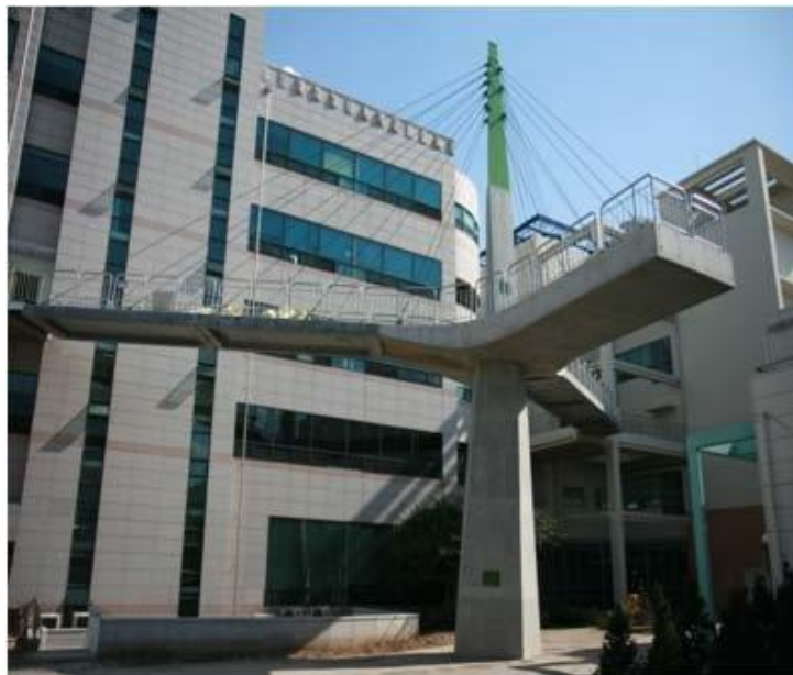
Fig.1.8: UHPC Girder Pedestrian Cable-Stayed Bridge (Source: www.researchgate.net )
