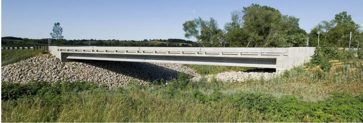
Fig.1.7: Mars Hill Bridge, Wapelo County, USA (Source: www.ductal.com )
