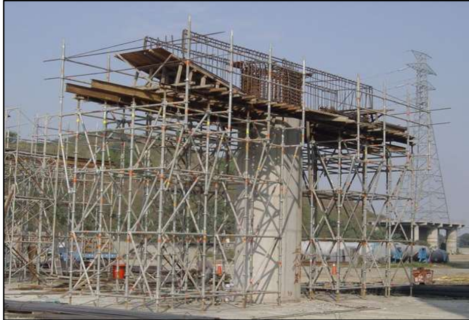
Figure1.1 Formwork for a wide Pier Cap, google
