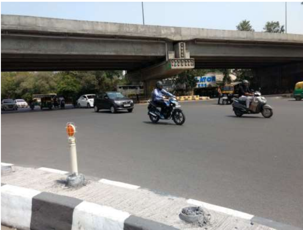
Figure1.4 Fully Prestressed Pier Cap, clicked by self
