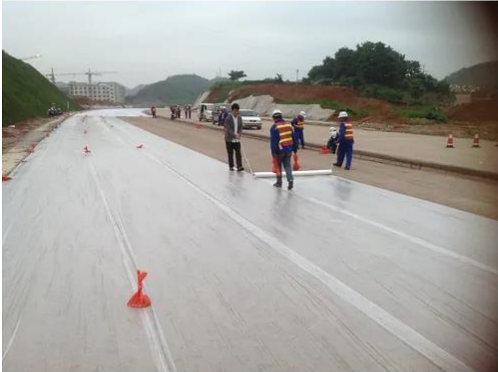
Fig 1.3: Membrane curing ( https://www.tradeindia.com/fp2329434/Concrete-Curing-Membrane-For-Road-Base.html )
