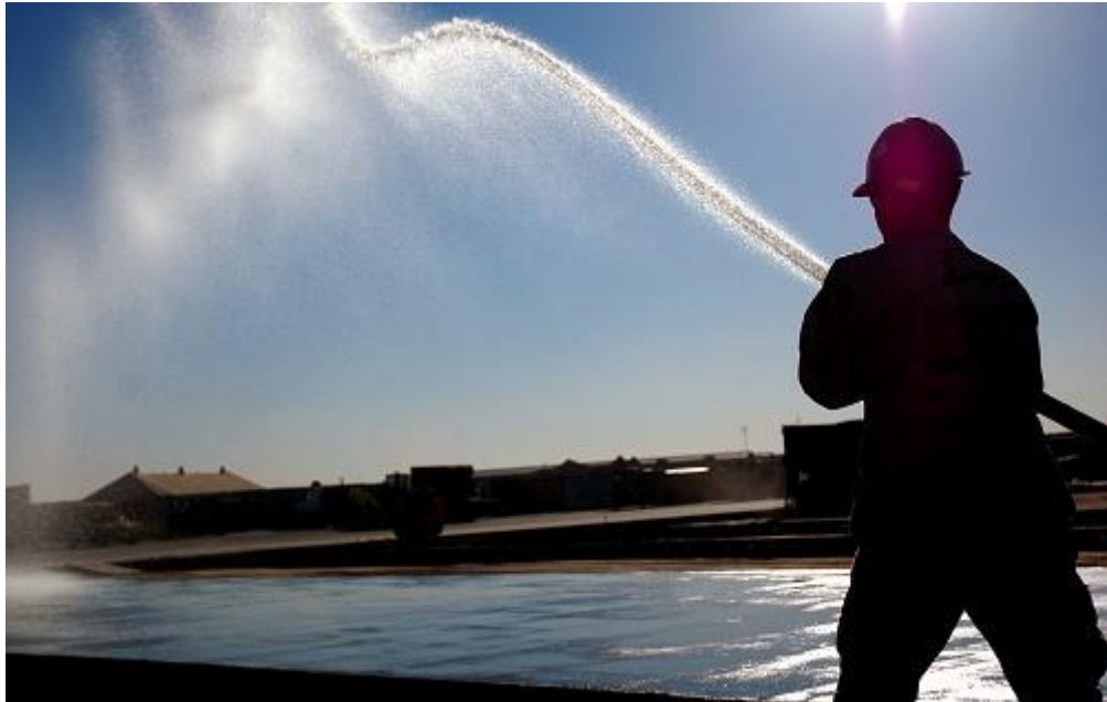
Fig 1.1: Sprinkling Water Curing ( https://blog.yellowpages-uae.com/methods-of-curing-concrete/ )
