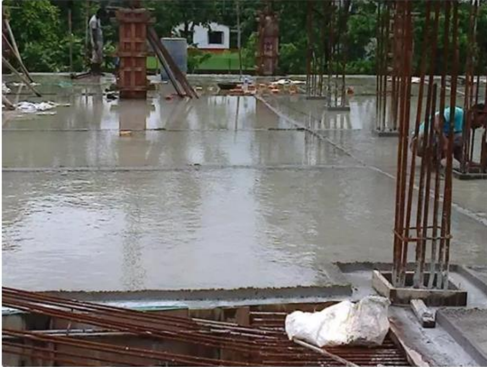
Fig 1.2: Curing by Ponding method ( https://www.quora.com/What-is-the-meaning-of-curing-in-civil-engineering )
