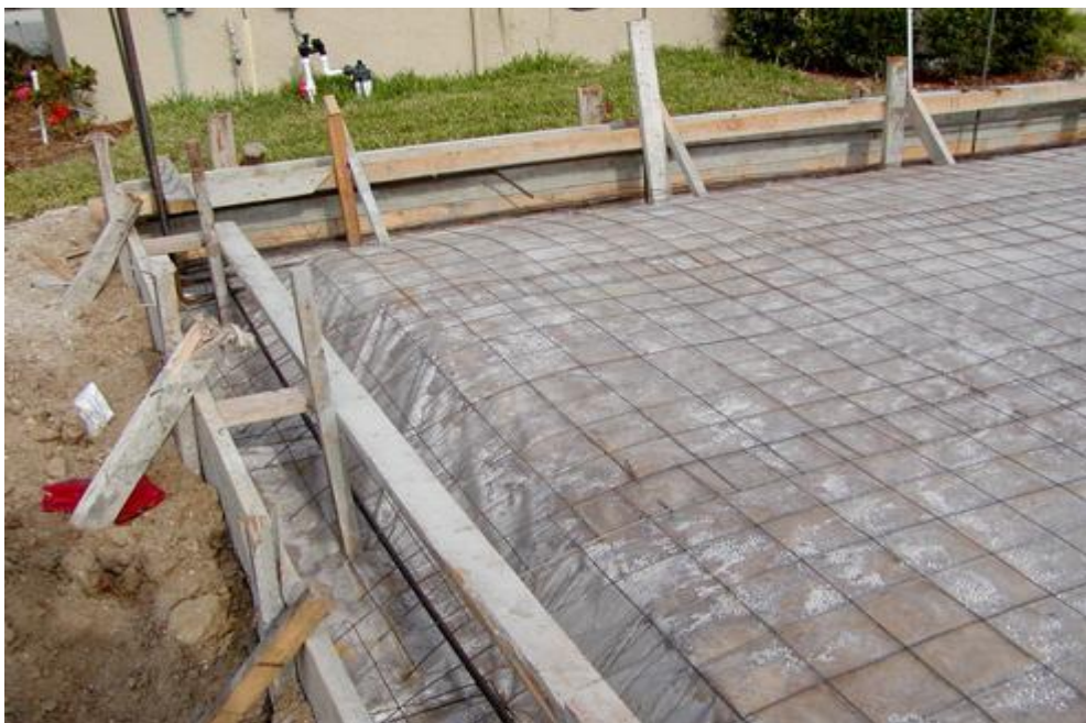
Fig 1.5: Sealed curing ( http://civilengineersforum.com/concrete-curing-methods-advantages-limitations/ )
