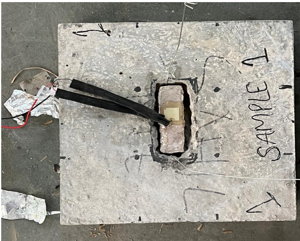
Figure 3. 13 Anode is placed in the Drilled area
