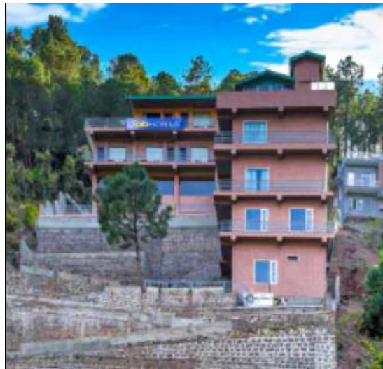
Figure 1.2: Building with Stepback columns in Himalayas
