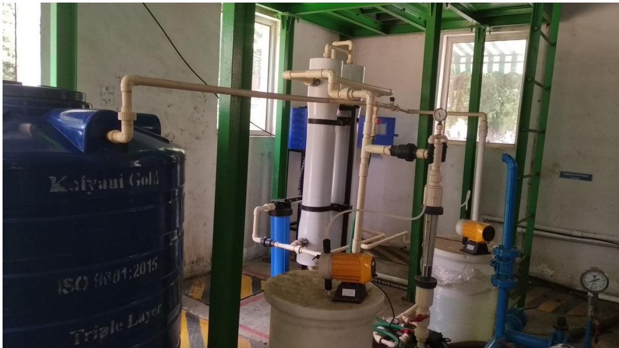
Figure 5.3: Present setup of Ultrafiltration unit
