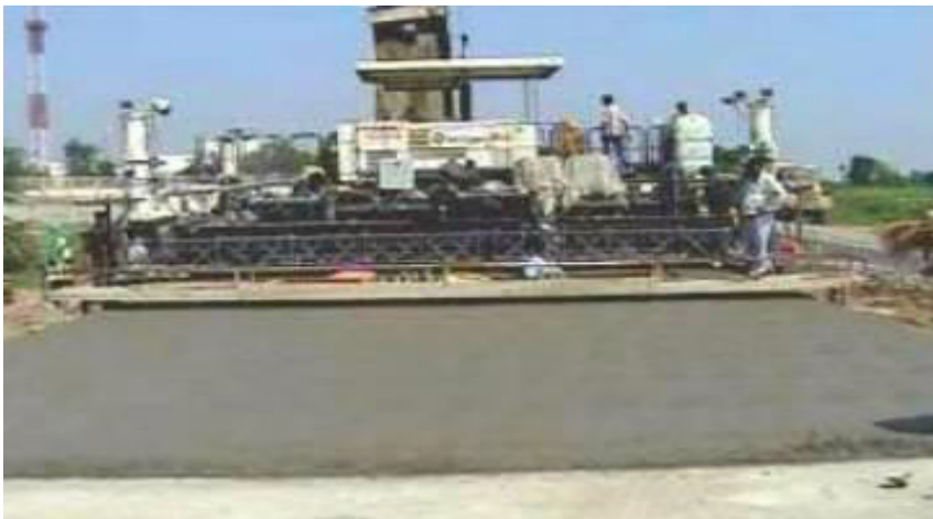
Figure 1.6: Construction of Concrete Pavement Slab With Slip-Form Paver ( NHAI, Kanpur )
