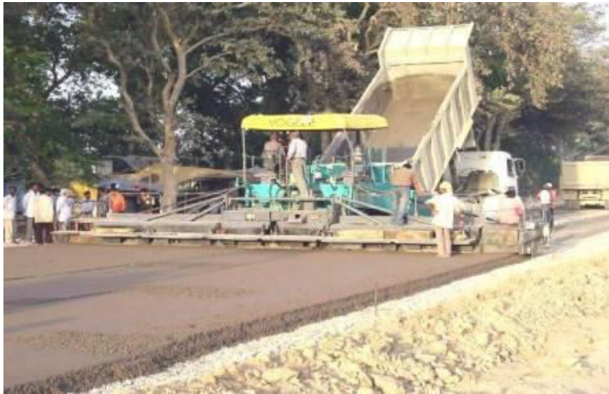
Figure-1.2: Laying of DLC ( photo NHAI, Kanpur )
