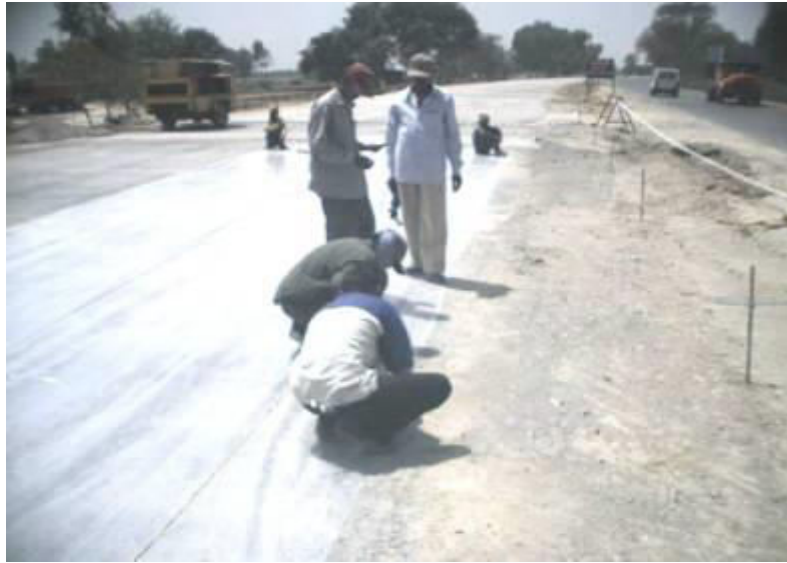
Figure-1.4: Laying of Polyethylene Sheet Over DLC ( photo NHAI, Kanpur )
