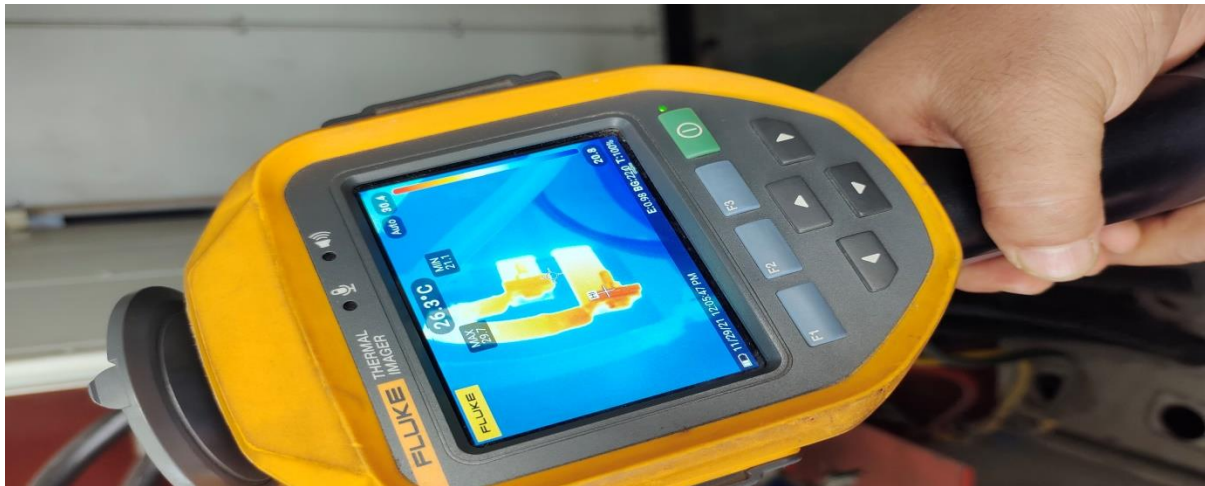
Fig. 5.6 Infrared camera used for various testing in the electrical facility
