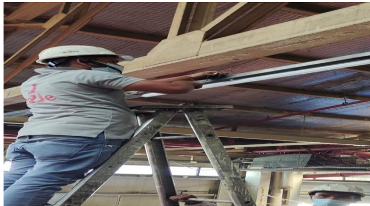
Fig. 4.10 working of manpower for some electrical works
