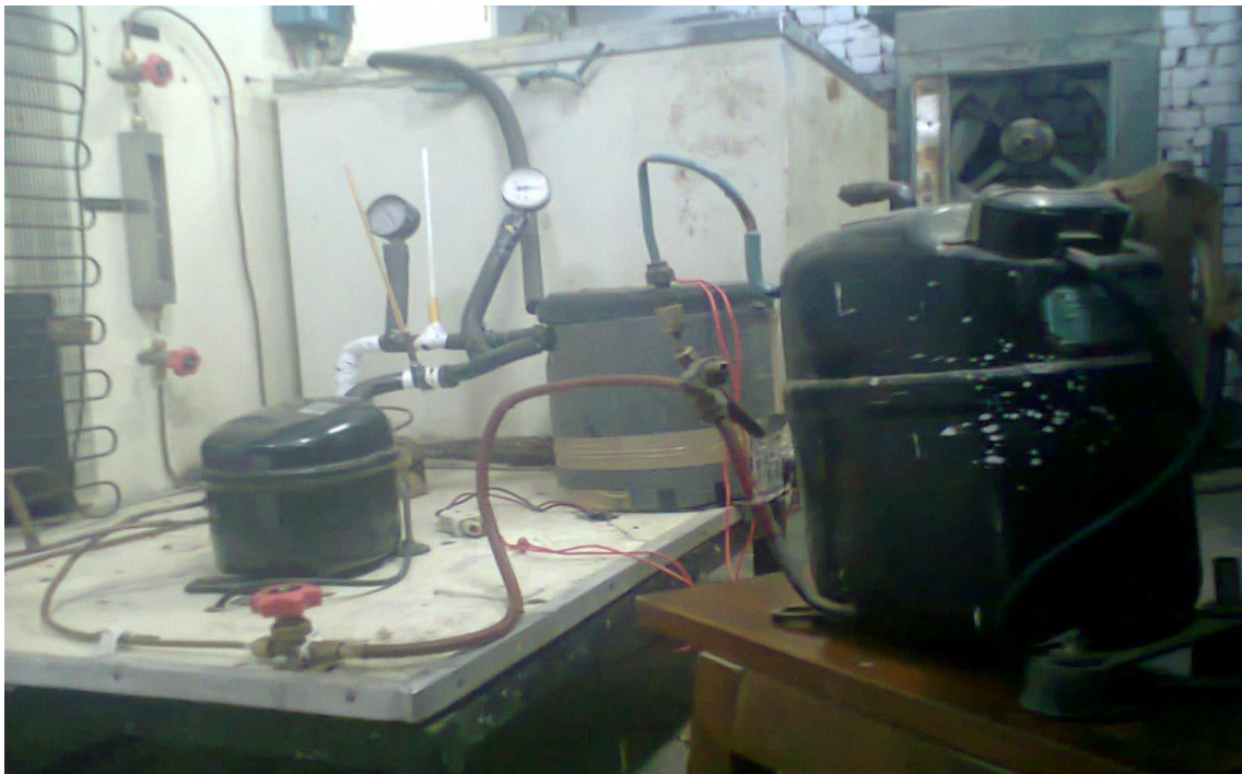
Figure 5.24: Vacuum compressor [RAC Lab, Thapar Uni.]
