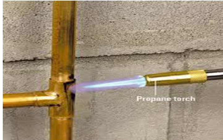
Figure 5.20: Silver brazed Tubing process [RAC Lab, Thapar Uni.]
