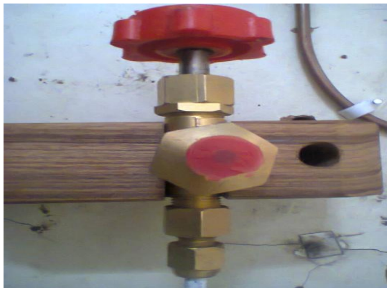
Figure 5.5: Handing operated expansion valve [RAC Lab, Thapar Uni.]
