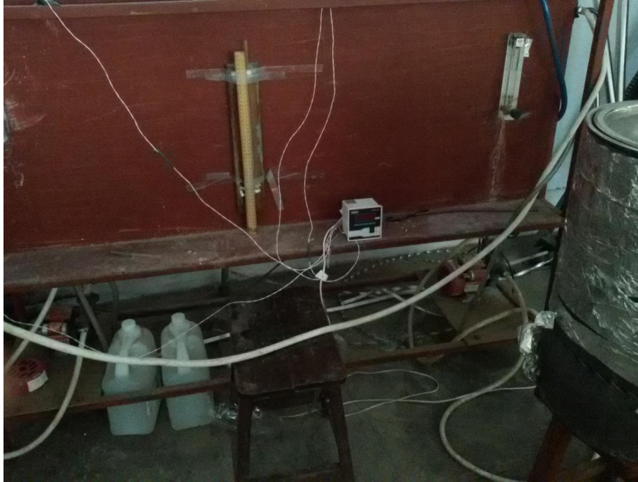
Fig 4.4.2 shows the working system of cold and hot water pipe in heat exchanger
