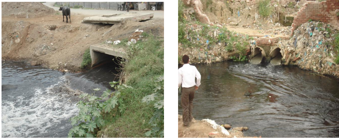
Figure 1.3: Outlets discharging effluent directly into the Nallah
