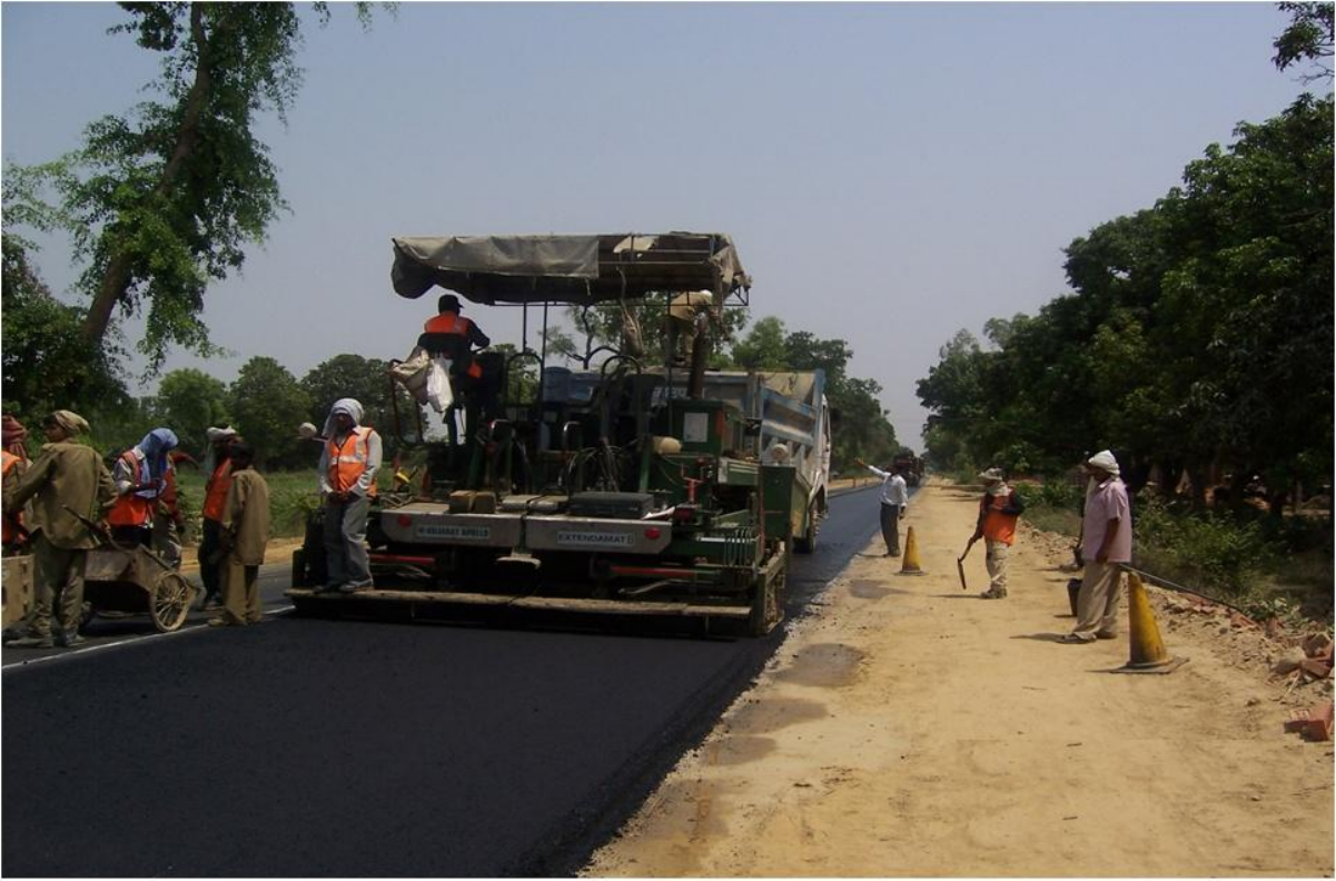
Plate 1.3: Laying of DBM mix at site.
