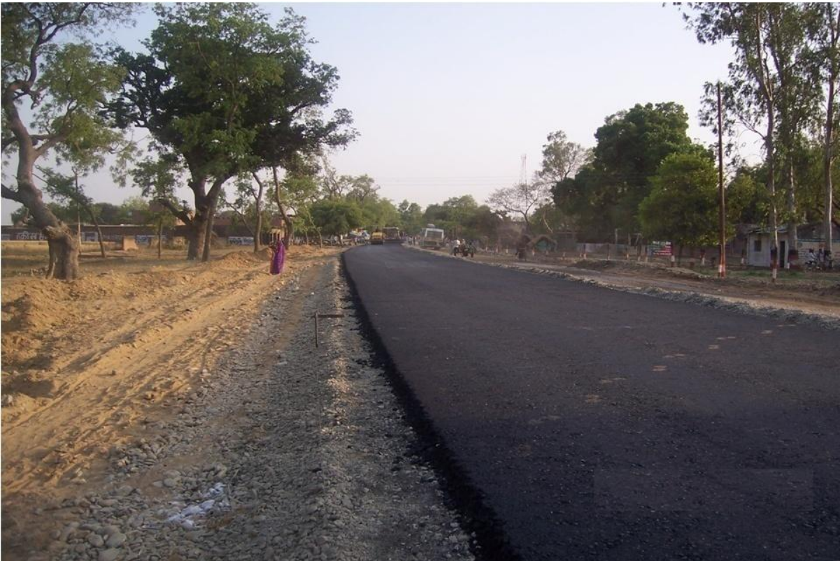
Plate 1.4: Final view of compacted layer of DBM
