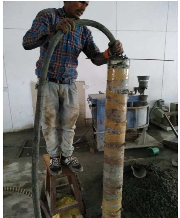
Fig 4.15: Needle vibrator for the compaction
