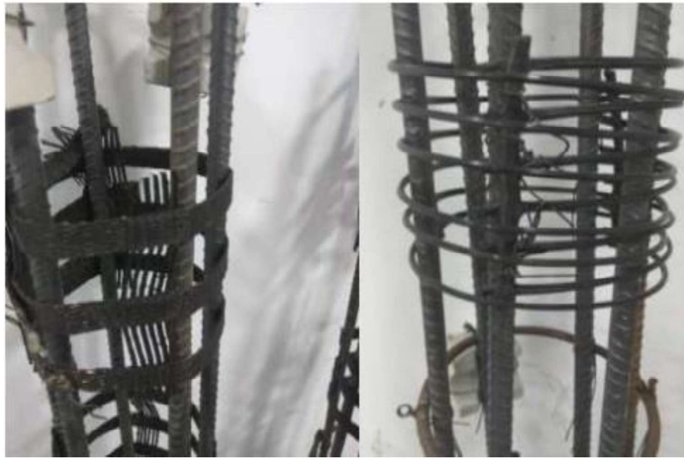
Fig 4.7: Applying geogrids on the sections.
