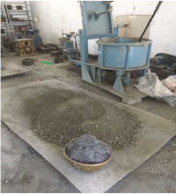
Fig 4.12: Dry hand mix of the concrete
