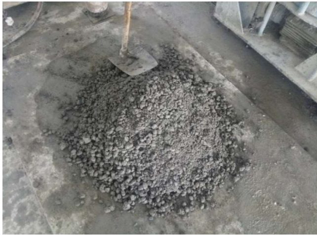
Fig 4.2: Hand mixing for normal concrete
