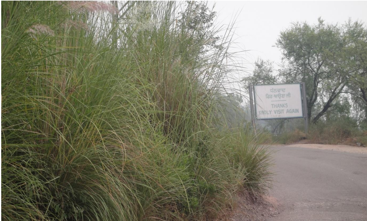
Fig 3.6 Curve with lot of sight obstruction and without any road signs and markings.
