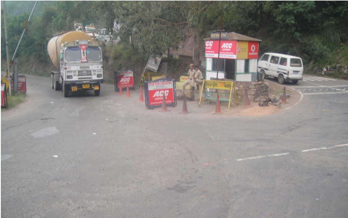
Fig 3.8 Improperly designed intersection without proper markings and sign
