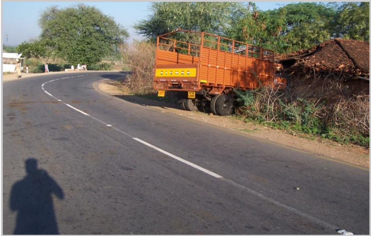
Fig 3.22 Accident on the horizontal curve
