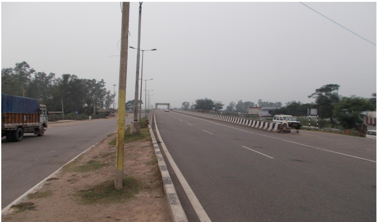
Fig 3.3 A four lane highway just before the start of project road
