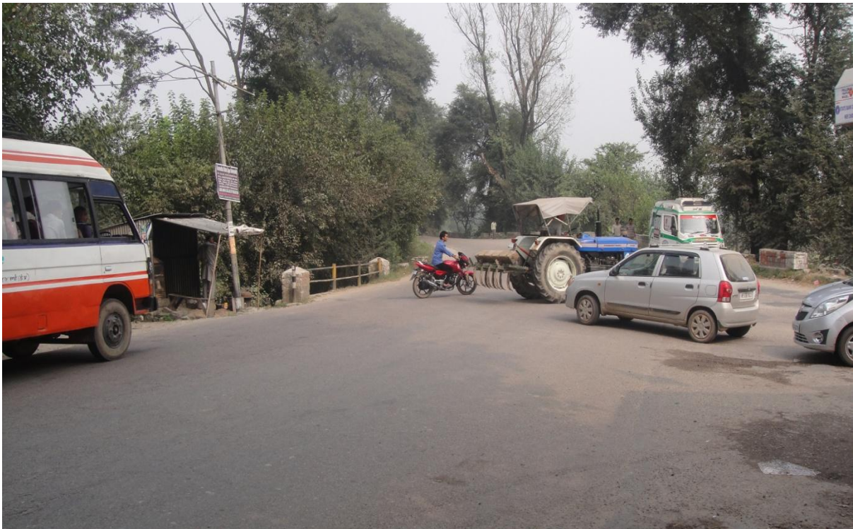
Fig 3.19 Improper Intersections without any safety aspects on the exiting highway.
