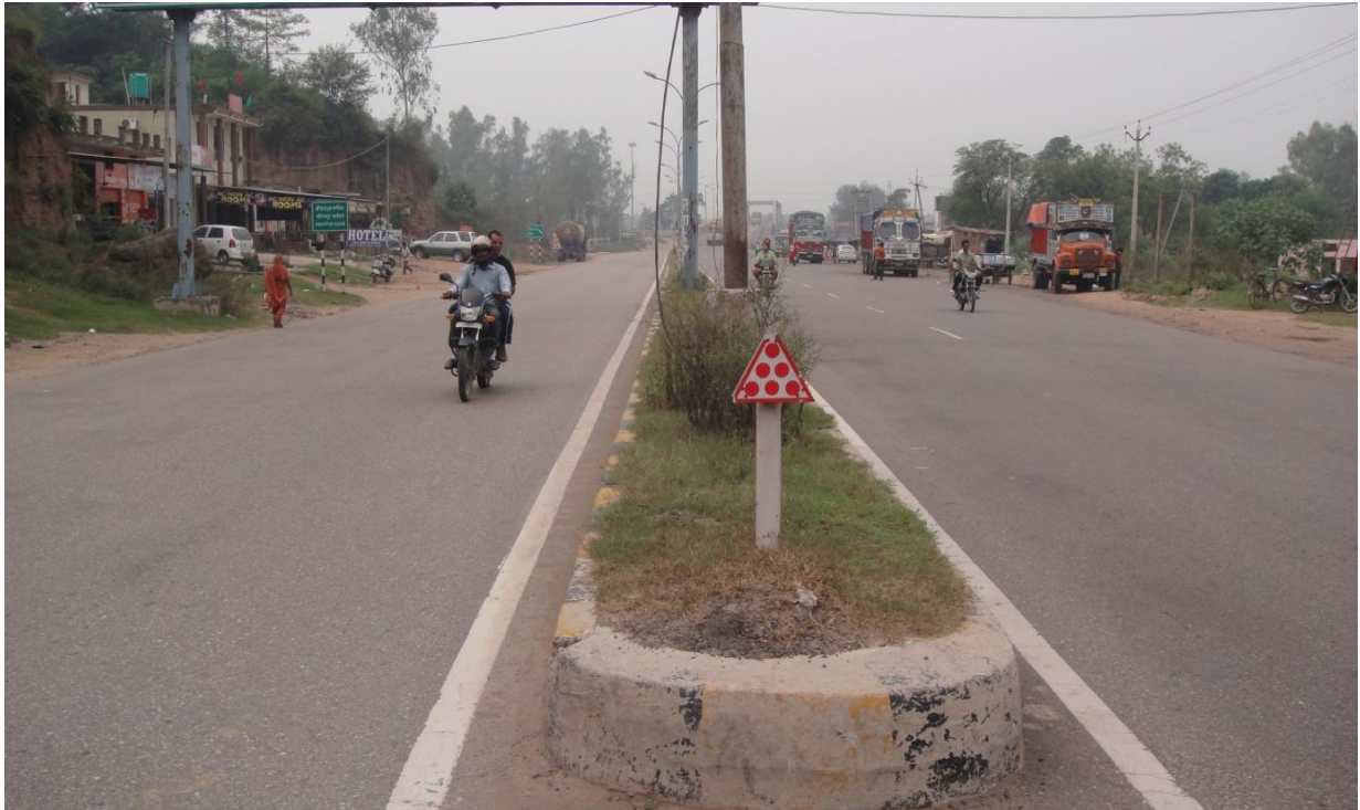
Fig 3.2 Start of the Project Site at km 73+200
