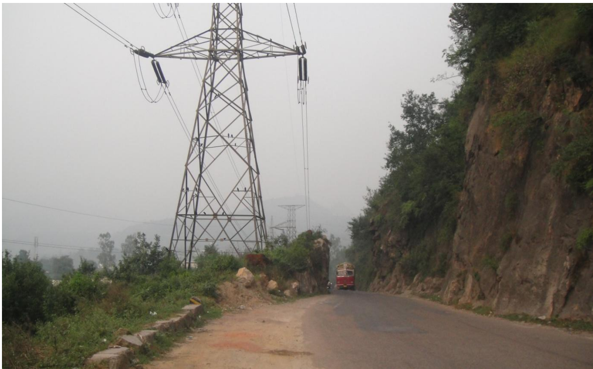
Fig3.11 Transmission tower on the road side without hazard sign and inadequate width
