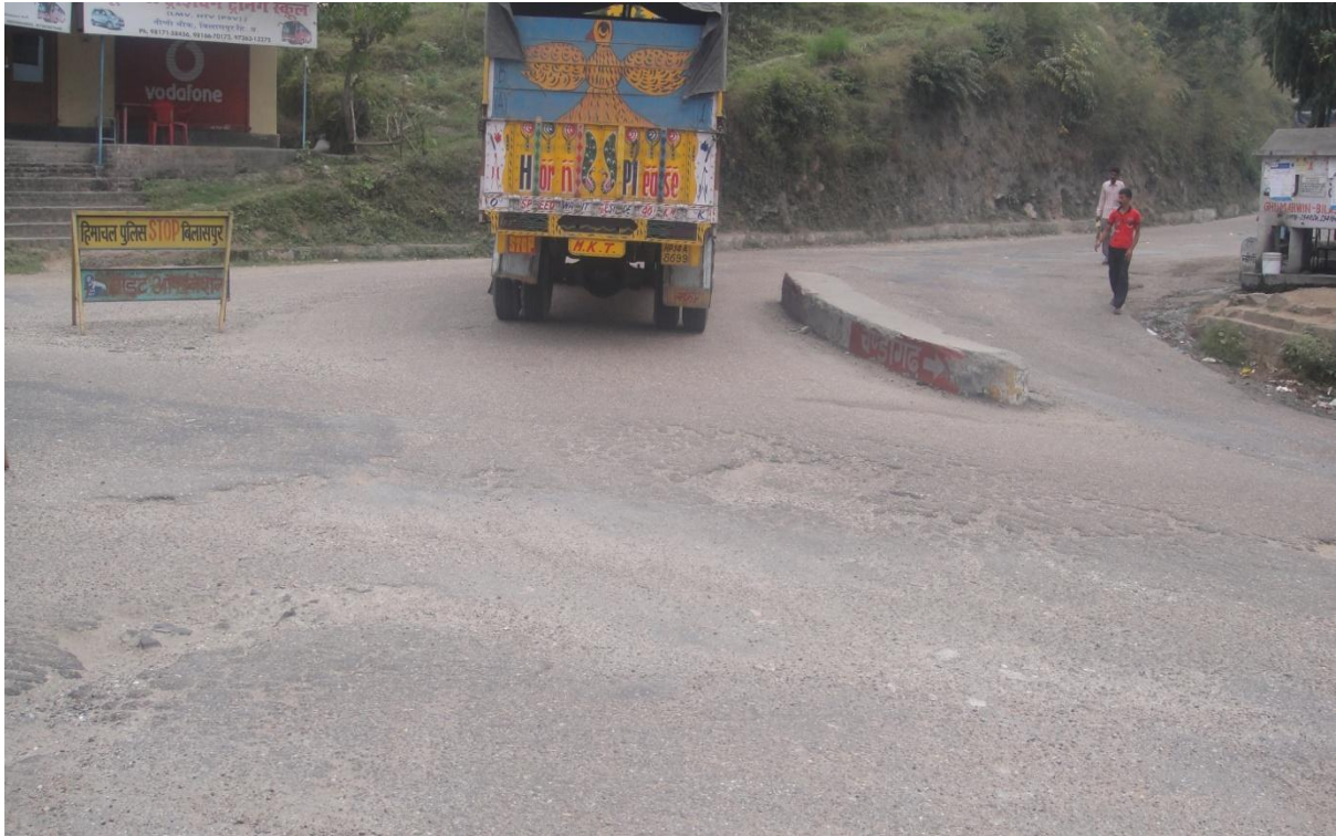
Fig3.10 Median with improper dimensions.
