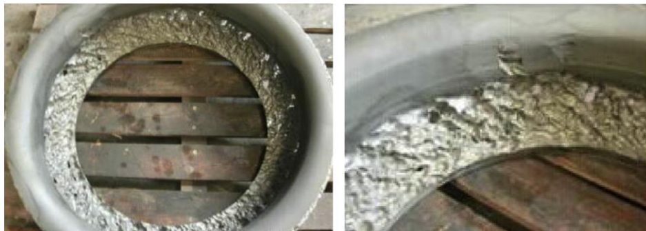
Figure 1.2. Erosion wear on shroud of slurry circulation pump at actual condition [Qiu et al. 2015, Electronic and printing permission of ©Elsevier].
