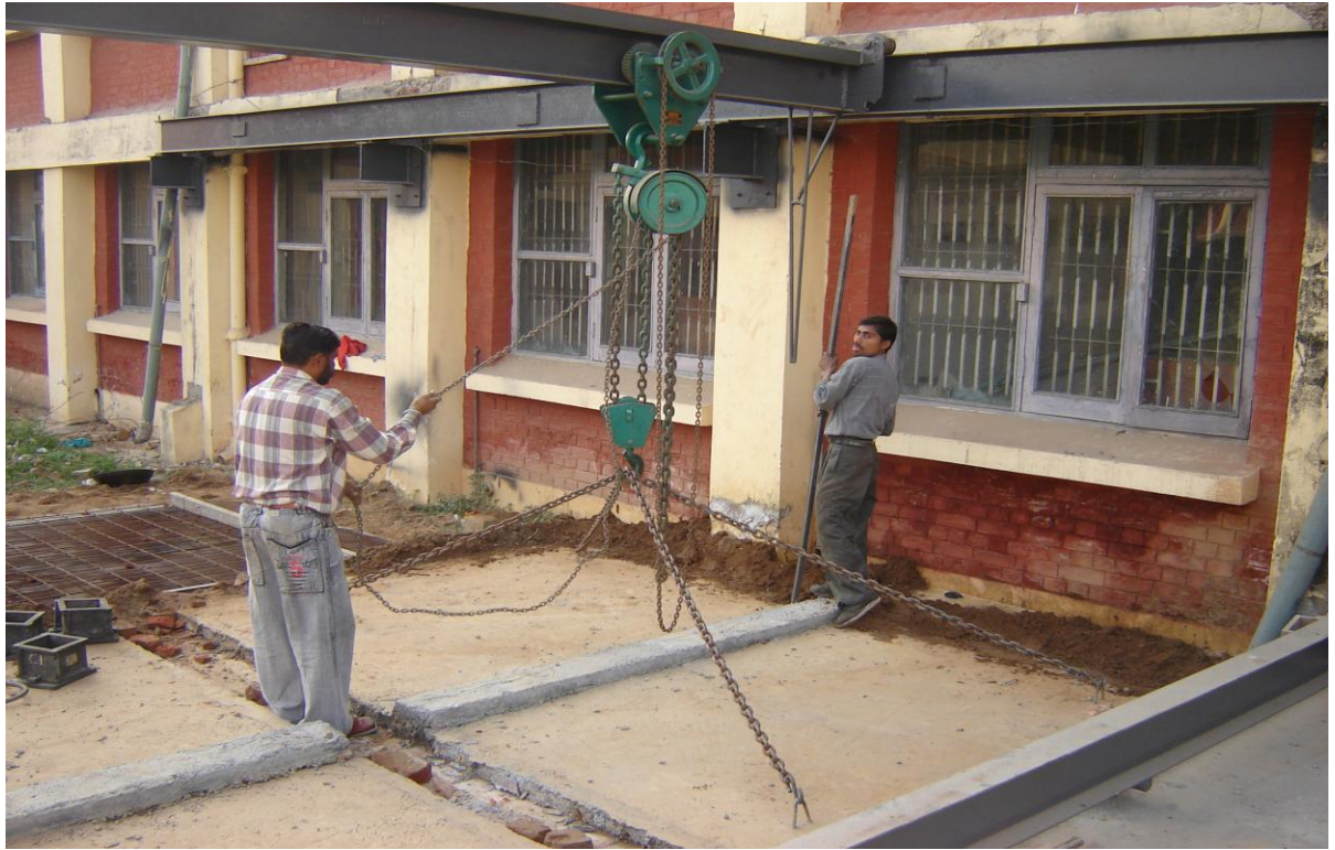
Figure 4.10: Typical Schematic Diagram showing the Lifting Operation of Slab
