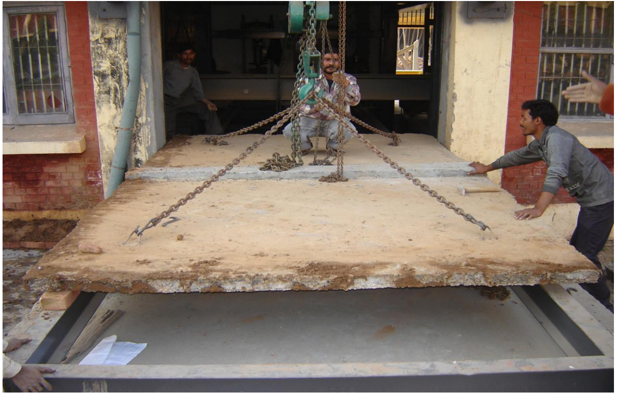
Figure 4.10B: Typical Schematic Diagram showing the Lifting Operation of Slab
