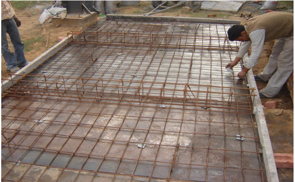
Figure 4.9B: Typical Reinforcement Detailing of 3-panel Slab
