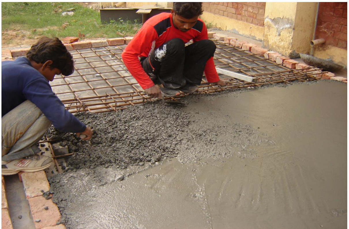
Figure 4.9A: Typical Schematic Diagram showing Casting of 2-panel Slab
