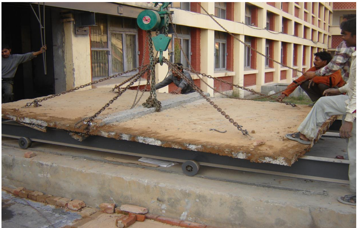
Figure 4.10C: Typical Schematic Diagram showing the Transferring Operation of Slab
